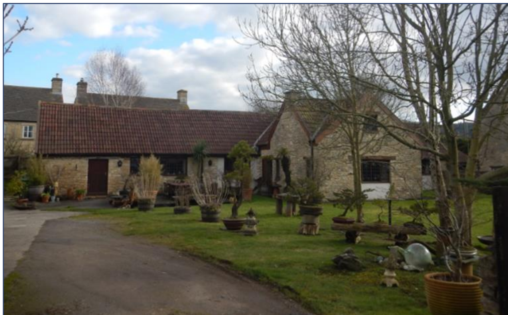
Figure 2: Photograph of dwelling at Longcroft Farm
