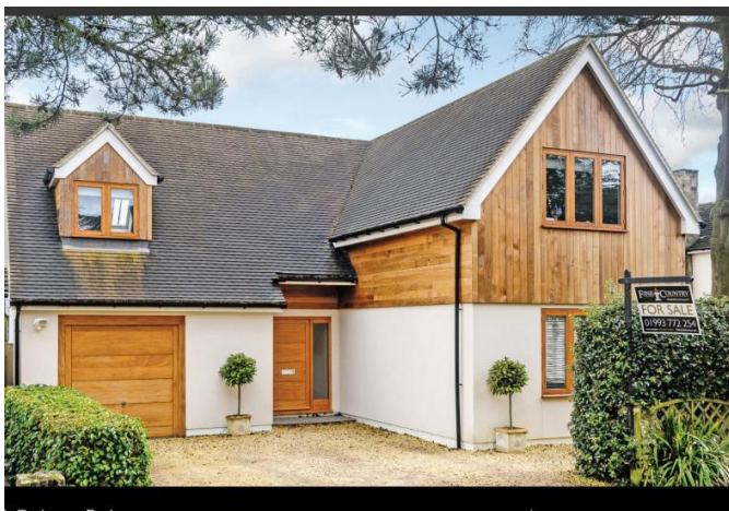
Photo 4 -6 Cadogan Park completed with 2 storey gable
