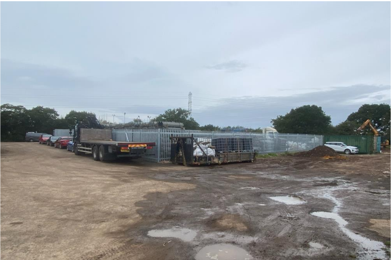
2 View from South East corner
