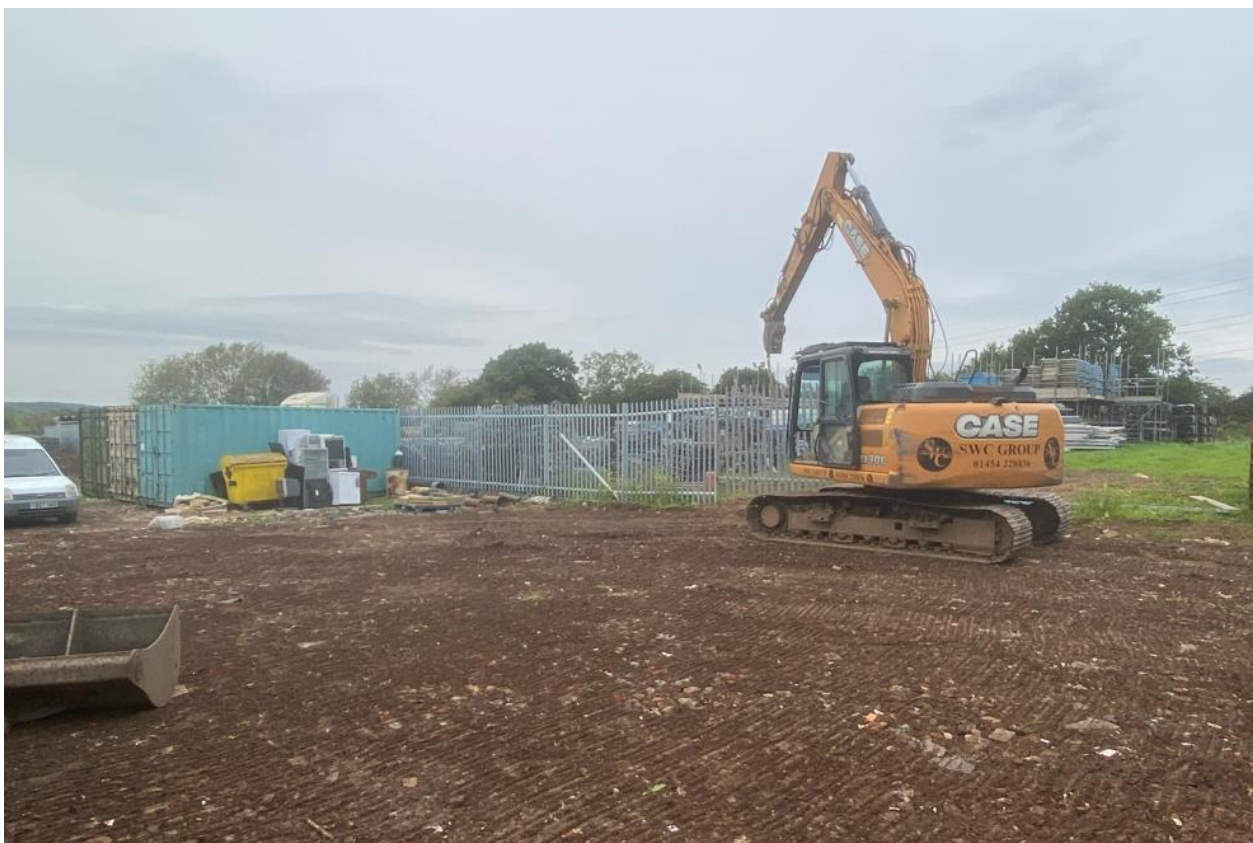
3 View from North East corner
