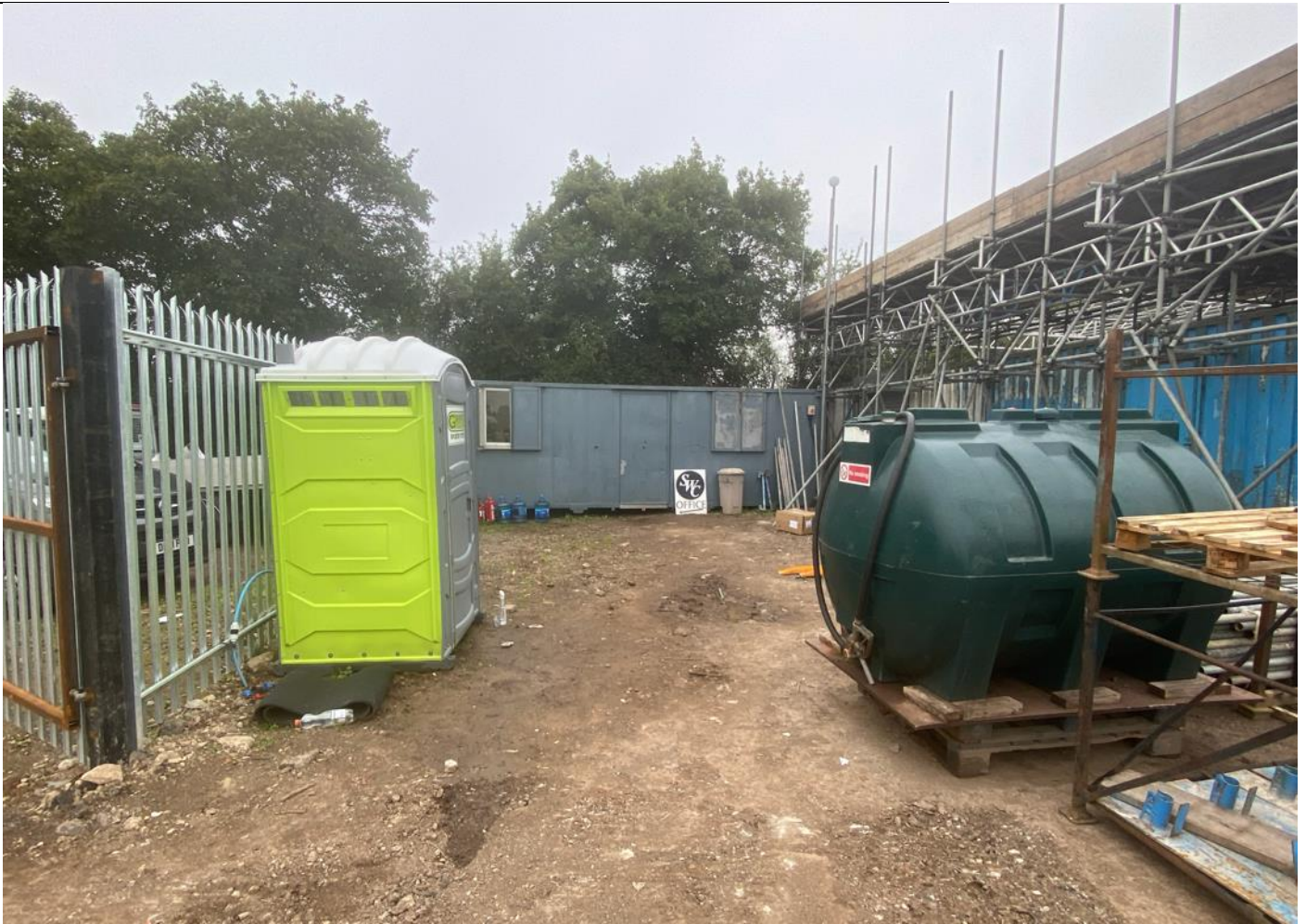
7 General view within yard – Site office and WC
