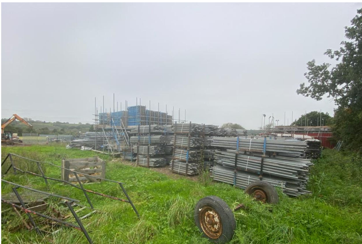
4 View from North West corner
