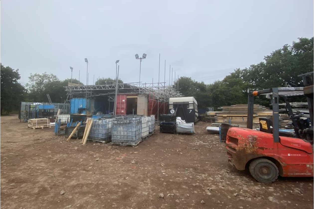
5 General view within yard – Looking West
