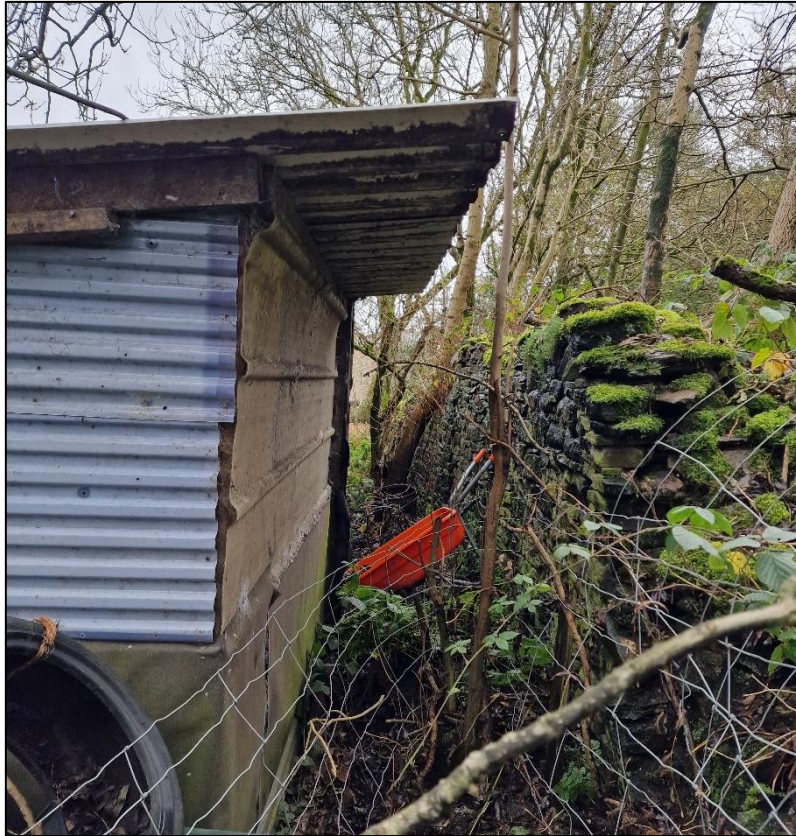
Plate 11 – The western face of B2, showing the dry-stone wall boundary
