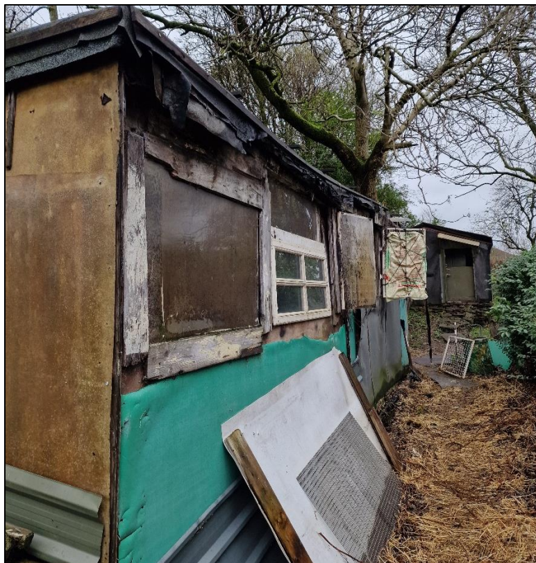
Plate 8 – Building 2 (B2) eastern face
