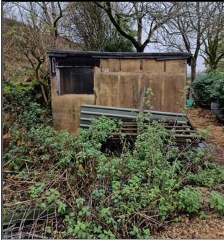
Plate 7 – Building 2 (B2) southern face with bramble scrub adjacent
