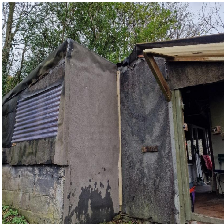
Plate 4 – Building 1 (B1) southern face
