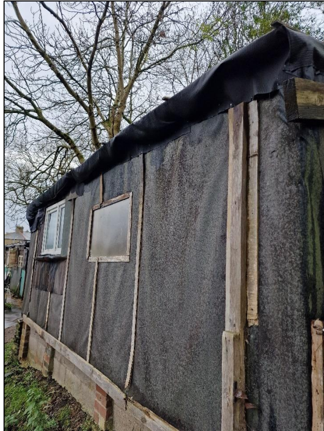
Plate 5 – Building 1 (B1) eastern face
