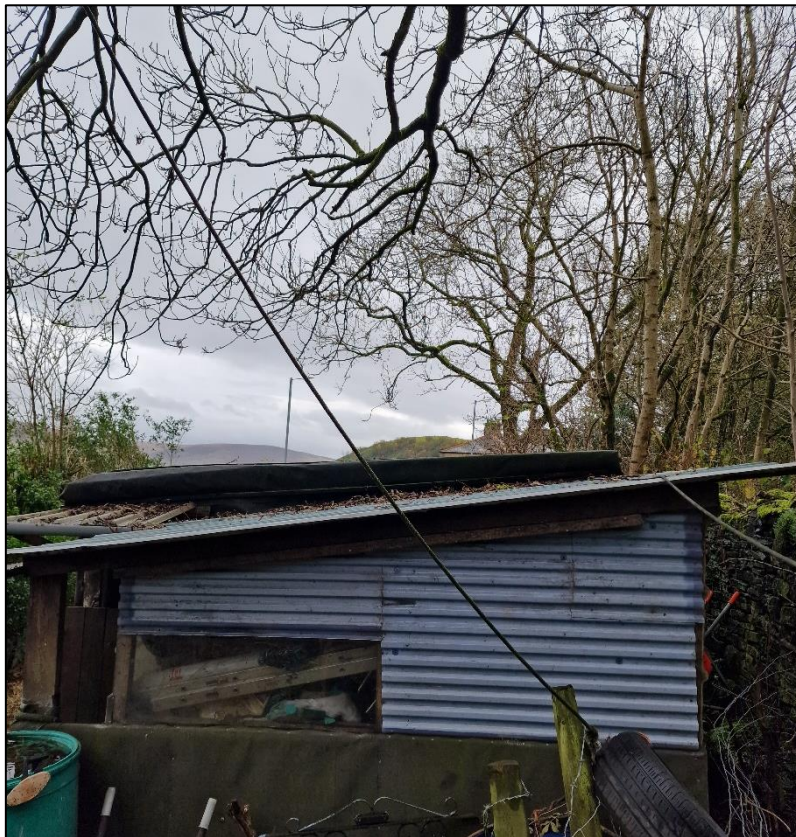
Plate 10 – Northern angle of B2 showing roof
