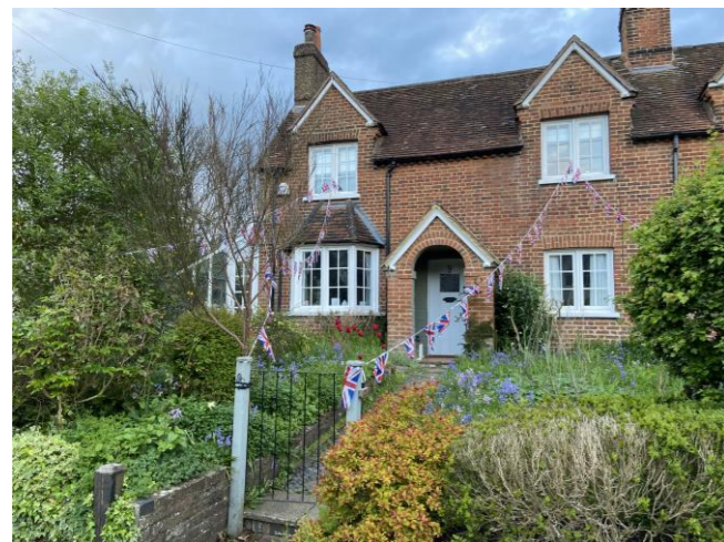
Image 3: View of No. 9 Solesbridge Lane
