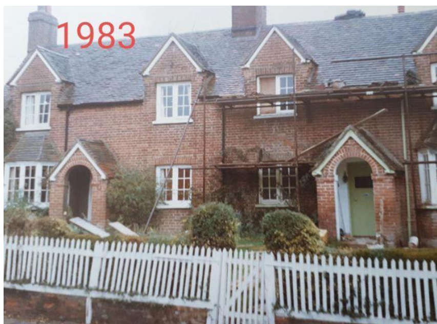
Image 3 Front Elevation to No. 9 & No. 10 Solesbridge Lane in 1983.
