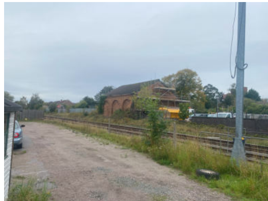
Fig 1.6 Photo Existing North West Elevation
