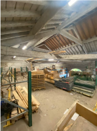
Fig 4.0 Existing Intricate Roof Structure
