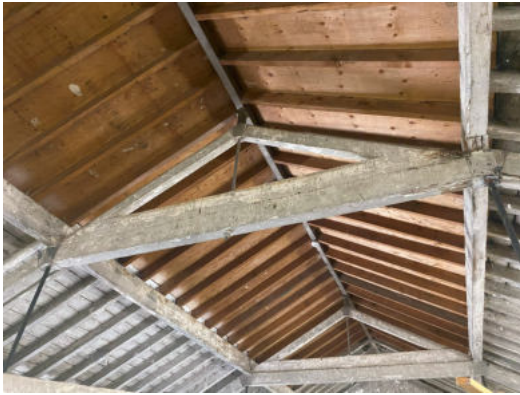
Fig 4.1 – Original Historic Rooflight location
