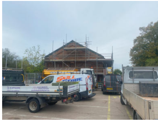
Fig 1.9 Photo Existing North East Elevation
