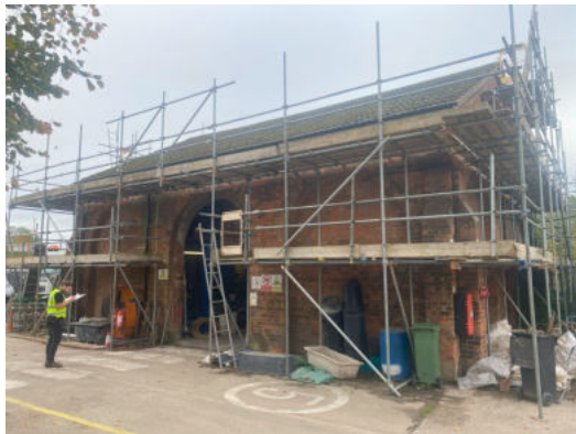
Fig 1.5 Photo Existing North West Elevation
