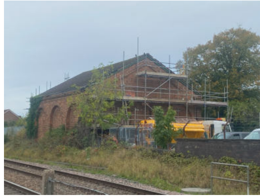
Figure 4.6 – View from opposite side of the Railway Line
