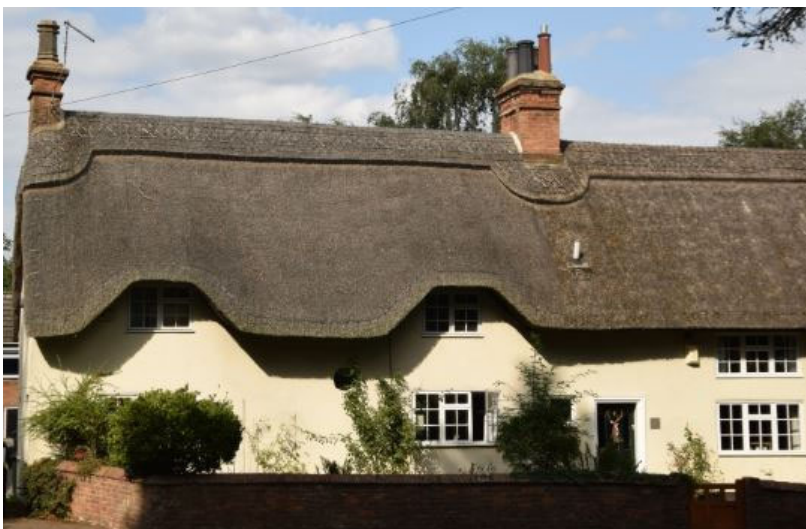
Fig 7. Church Court Farm
