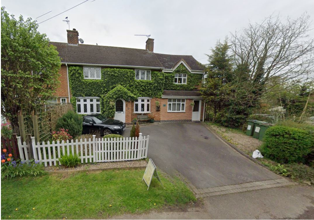
Fig 4. Street scene - No. 7 Hinckley Road
