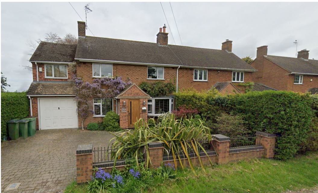
Fig 3. Street scene - No. 13 and 11 Hinckley Road
