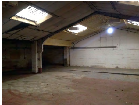
Interior of asbestos clad barn
