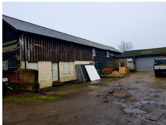
Fig.02: Barn rear and stock yard
