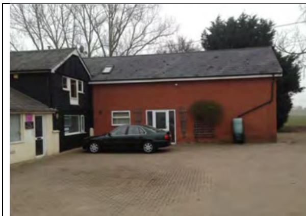
Photo ref 1. Eastern edge of mid-section of buildings (also showing eastern annexe). All buildings previously onsite have been demolished.
