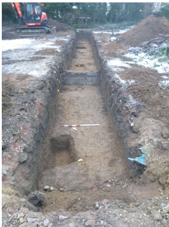
Photograph 3 T3 trench shot – looking northeast
