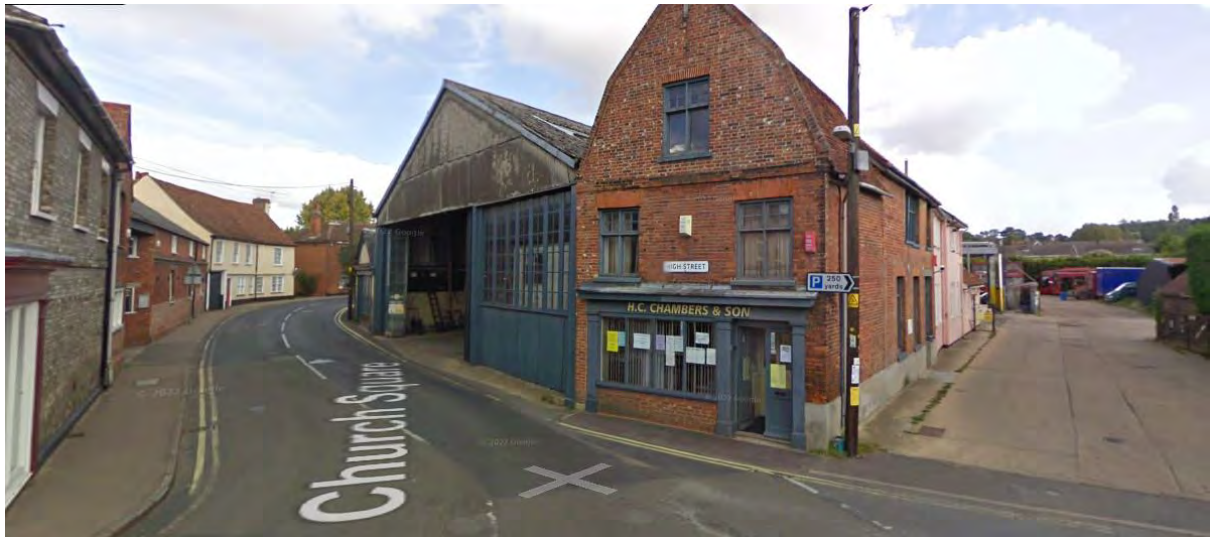
Plate 2-6: Depot buildings and site access in September 2011 (source: Google Streetview)
