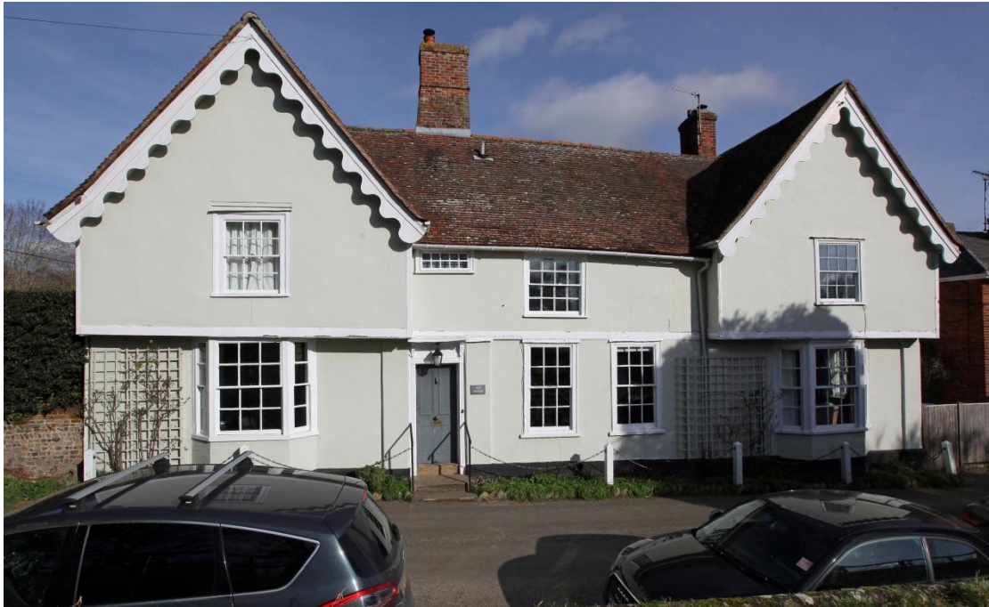
Illus. 1. The picturesque south-western facade showing the barn-like open hall in the centre with the jettied parlour cross-wing on the left and the matching service wing to the right. The original cross-passage lay to the right of the hall and probably under the service jetty but was later replaced by a lobby entrance in front of the inserted chimney which heated both the hall and parlour. This chimney was largely or wholly rebuilt along with the brick ground-floor walls as part of a major mid-19 th century refurbishment that included the reeded door case, sash windows and barge-boards.
