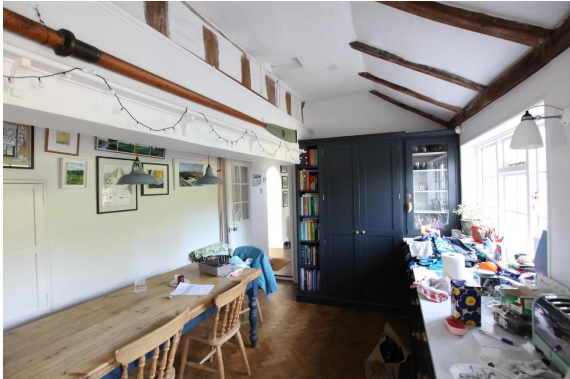
Illus. 13. The north-western end of the kitchen showing the modern machine-sawn false rafters to the right and the original weathered external studs of the open hall to the left. The lower section of the hall has been removed to enlarge the kitchen and the surviving studs and post are presumably supported by a hidden RSJ. The false roof-plate and rafters of the lean-to were inserted beneath the sloping plaster ceiling to create a semblance of age, but the original rafters survive above (illustration 16).
