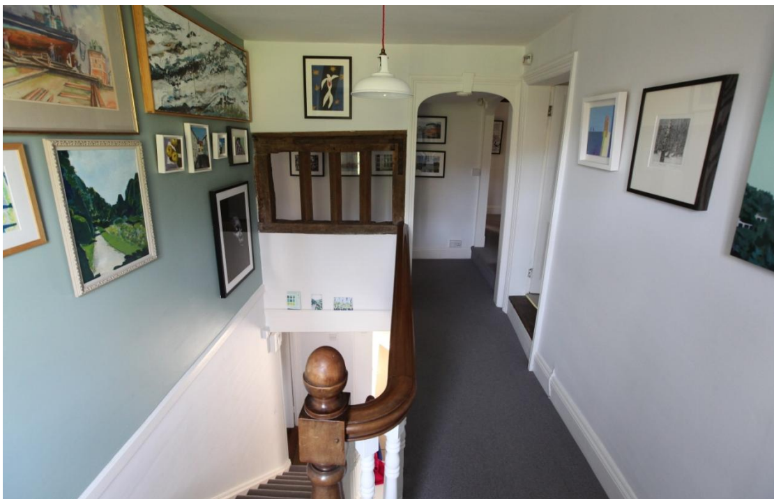
Illus. 18. The first-floor stair landing from the rear, showing the heavy moulded mahogany rail of the Victorian stair in the foreground and the modern mullions of the medieval hall window in the rear. A tight spiral stair of the 17 th century is likely to have occupied the smaller turret depicted in 1838 which was later extended to accommodate the present stair.
