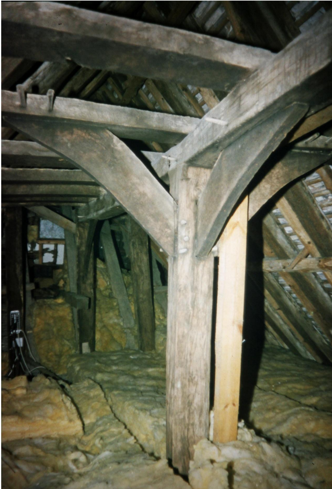
Figure 11. The plainly chamfered and step-stopped crown-post of the central open hall, as photographed in 1999 from the high end to the north. A modern pine plank has been inserted alongside, and the wattle-and-daub infill of the low-end wall in the rear has been removed to expose the rafters of the service cross-wing. The rafters and other original timbers are all evenly but lightly sooted, suggesting an open hearth was replaced by a chimney within months rather than years.
