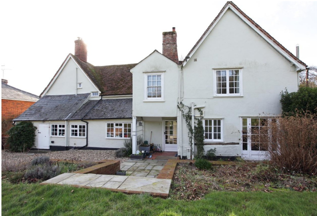
Illus. 3. The equally picturesque rear elevation with the slate-roofed lean-to additions behind the service wing and hall on the left. The three-bay parlour wing on the right contained an additional room that projected behind the hall and is now adjoined by a stair turret that was extended or rebuilt to accommodate the present staircase as part of the mid-19 th century refurbishment. The position of this turret is typical of the 17 th century but it is unclear whether any older fabric survived its extension.
