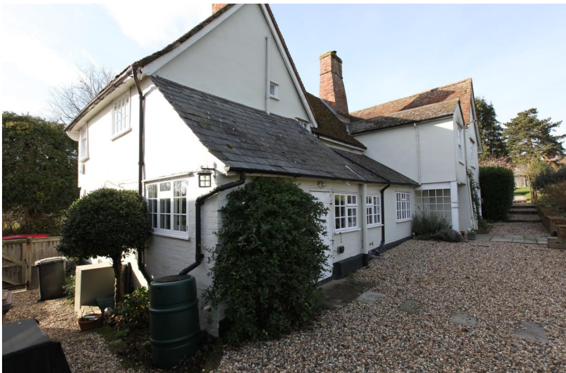
Illus. 4. The house from the south-east showing the painted brick fabric of the slate-roofed lean-to which appears to be integral to the lower storey of the service wing. The projection of the stair turret and parlour wing in the rear is just as depicted in 1884.
