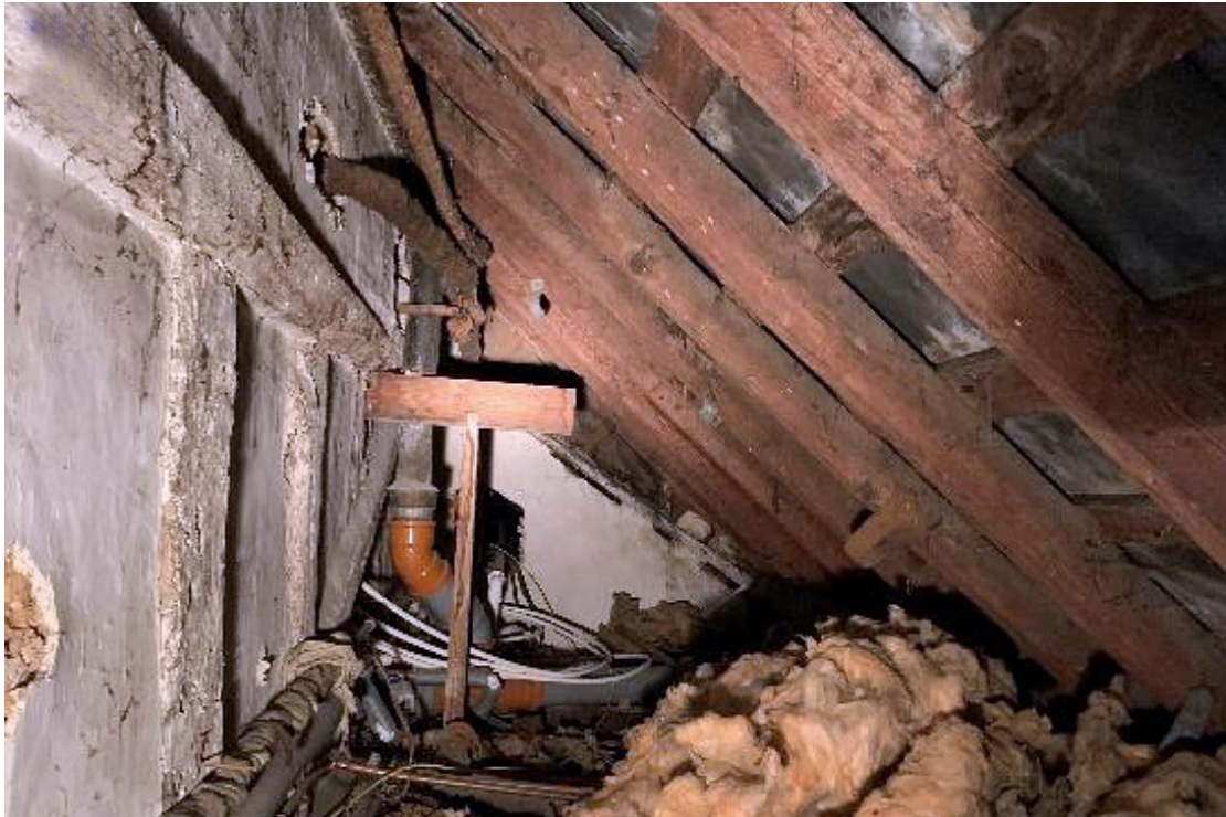
Illus. 15. The south-eastern end of the lean-to above the ceiling in illustration 10 (photographed by Odette Robson for her Bat Roost Assessment of March 2023). The roughly hewn hardwood rafters in the rear are typical of the mid-19 th century and the machine-sawn pine example on the right is presumably a replacement. Unless both the rafters and ceiling joists are secondary, the whitewash of the service wing's gable on the left was exposed externally prior to the lean-to construction.
