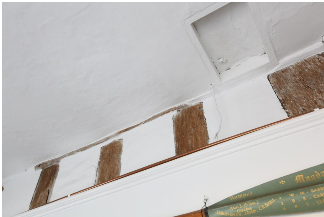
Illus. 14. A detail of the weathered studs of the hall's rear wall to the left in illustration 13 showing the nailed rail or clamp supporting the ceiling joists in illustration 16. The undulating lath-and-plaster ceiling is an original mid-19 th century feature.
