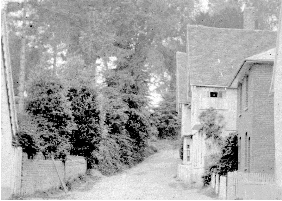
Figure 9. An early-20th century image showing a good 18th century casement window with leaded lights above the jetty of the service cross-wing. This has since been replaced by a sash window to match those of the street facade but probably indicates the building's appearance when acquired by William Synnott.
