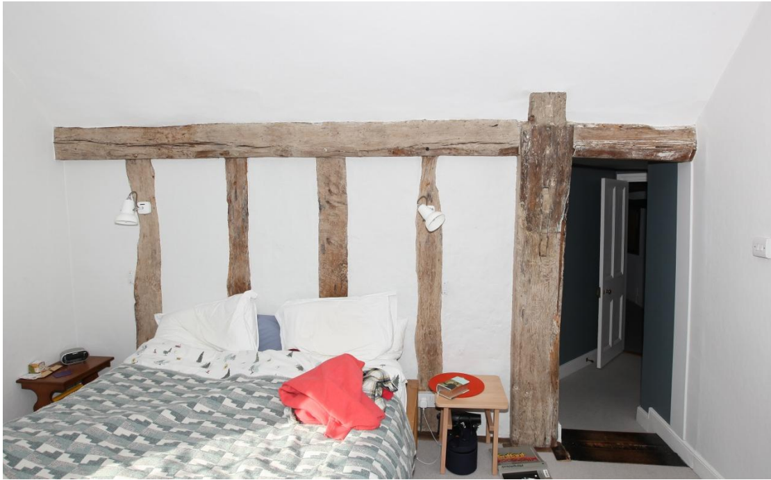
Illus. 9. The relatively widely spaced studs of the service cross-wing which are exposed in the first-floor wall of the service chamber adjoining the hall. A mortice for a high arch-brace to a missing tie-beam is visible in the jowled post alongside the present door. This is one of few areas of wall fabric currently exposed in the house and reflects the framing of the front wall (as indicated by the pattern of stud pegs in the hall's roof-plates and the parlour wing's exposed tie-beam). Many merchants' houses of the same period in Nayland contain expensive 'close-studding', with infill panels of no more than six inches, but the builder of Hill House focused on scale rather than ostentation.
