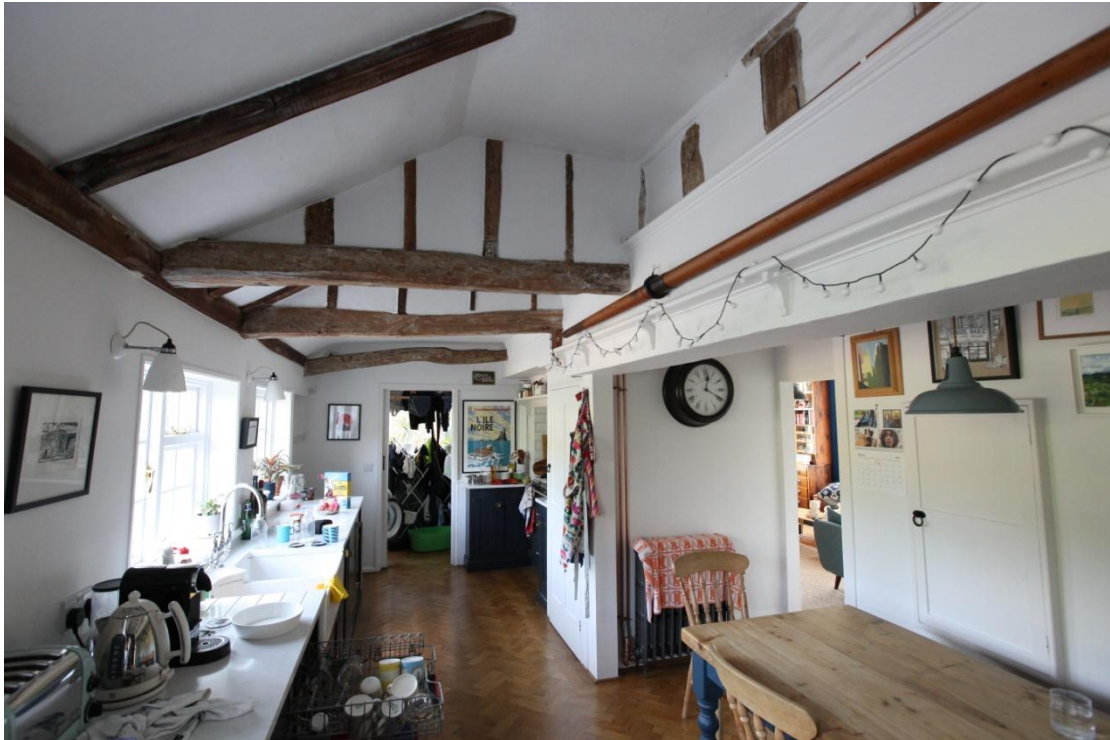
Illus. 11. The lean-to rear kitchen from the north-west. Little historic fabric is visible internally, with the brick wall on the left concealed by modern plaster. The three tie-beams in the rear are original features, as are most of the vertical studs above, but the exposed roof-plates and rafters are modern replicas. The window on the left is flanked by the tie-beams of former partitions suggesting it occupies the position of an original external door, although there is no obvious evidence of this in the external brickwork.
