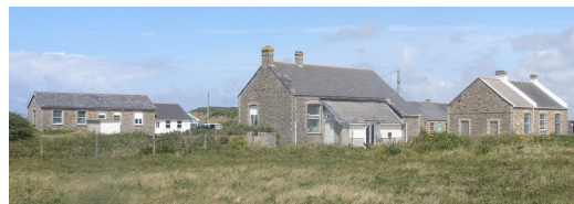
Plate 6 Site 18 office (centre), with Site 19 stand-by feeder plinth (left) largely covered with vegetation, looking northeast
