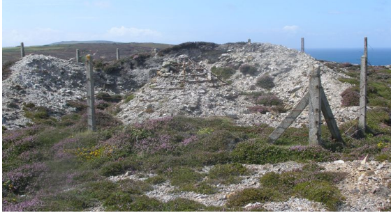
Plate 1 Site 1 shaft with collapsed collar looking west
