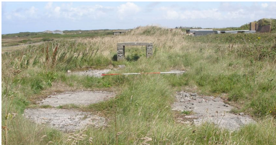
Plate 2 Site 4a Latrine and drying room floor with Site 4b concrete water tank stand in background, looking northeast
