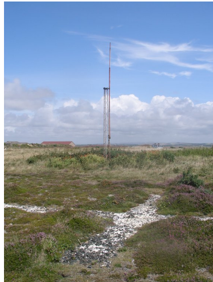
Plate 5 Site 12g landing marker (foreground) and 12f radio mast (rear) looking east
