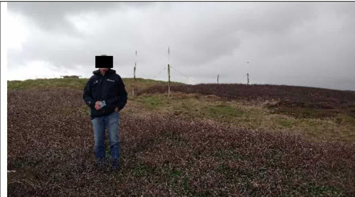
Fig 8 position of first set of new transmitter antenna
