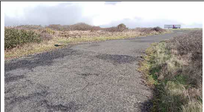
Fig 4 tarmac road within the cable run
