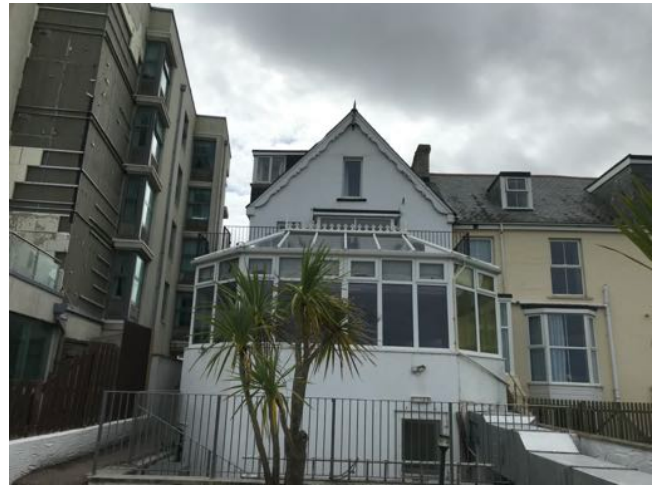
Image 2: Rear view of the main building.
