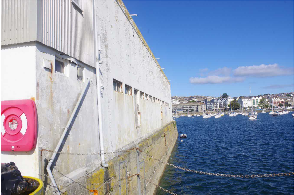
Fig 20 The Rank Building (Site 9), north east elevation.
