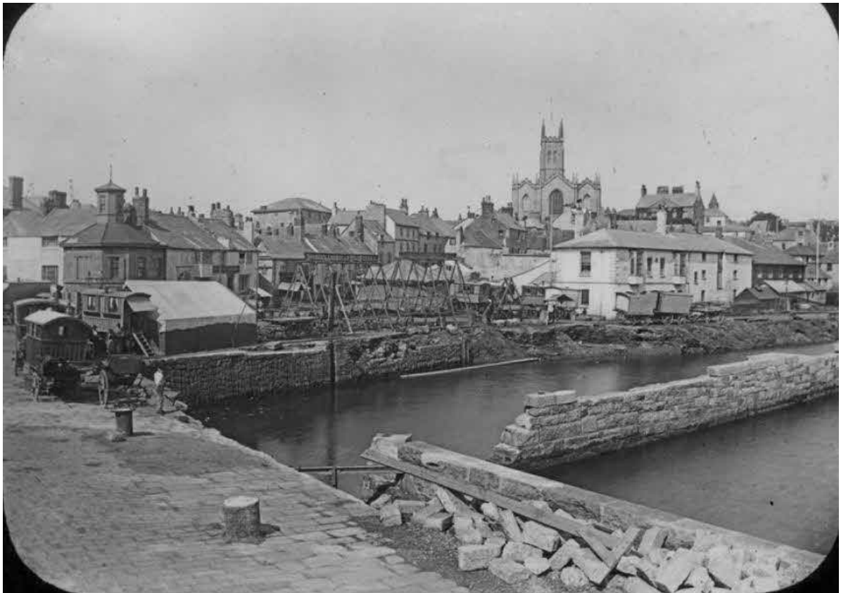
Fig 10 Construction of the floating dock c1879 © Morrab Library Ref: M.0260.
