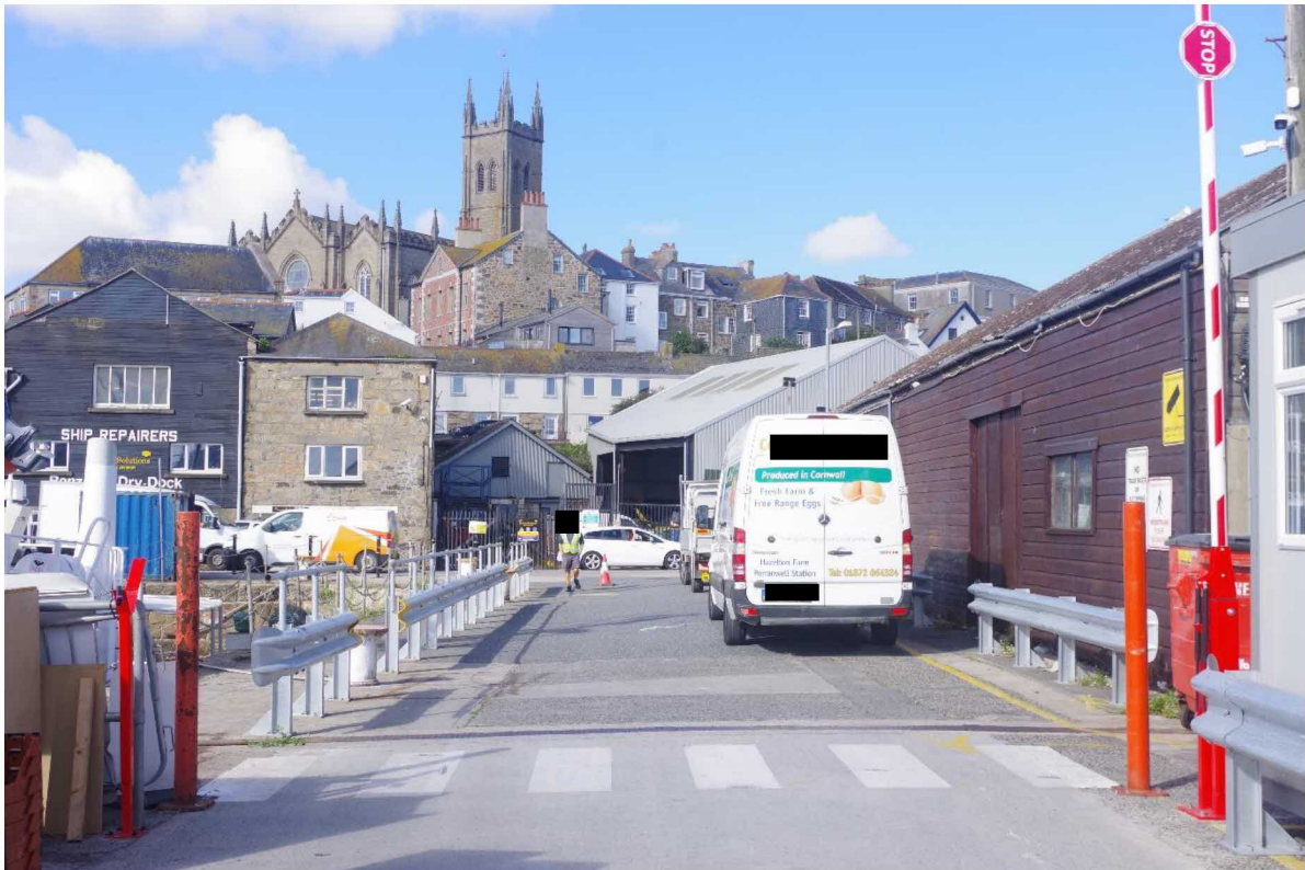
Fig 18 View along the western part of the North Pier (Site 1) looking towards the historic bonded store (left), the Grade II Listed dry dock (centre) and St Mary's church (Grade II* Listed) above.
