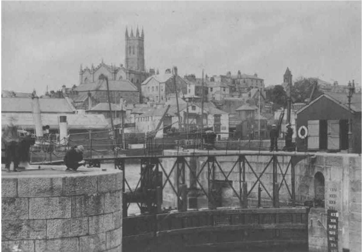
Fig 12 Floating dock gates taken in 1890-1900 showing dockside building on the western quayside (now Penwith Marine Services building and Boston building) © Morrab Library Ref: M.0177.
