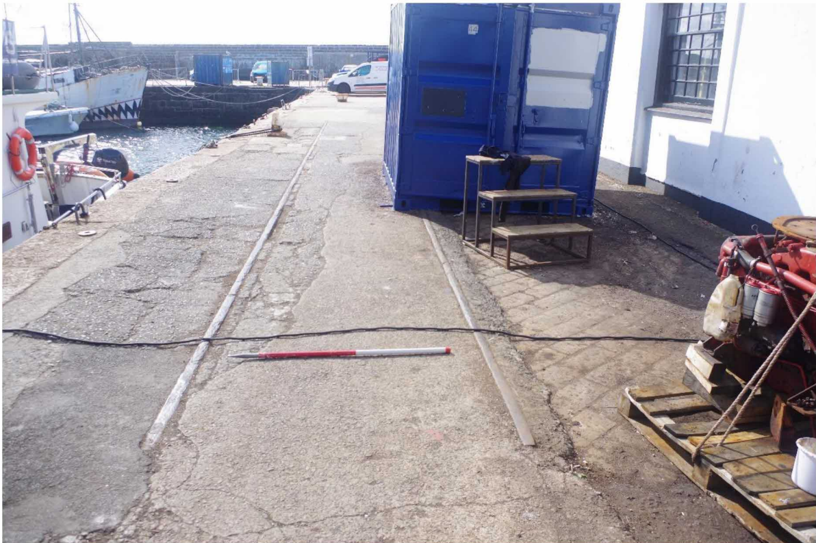
Fig 31 Tram rails and surface of granite setts (right) dating to c1880 (Site 38) outside the Waterside Meadery.
