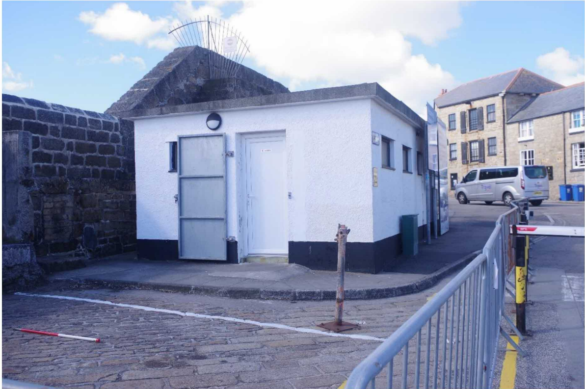
Fig 28 Historic, granite surface and modern toilet block at the western end of the Grade II* South Pier.
