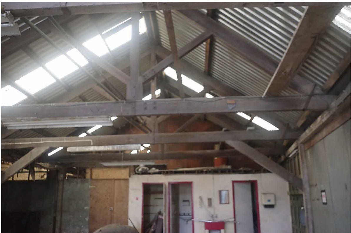
Fig 25 King post trusses dating to c1880 inside the Boston building (Site 34).
