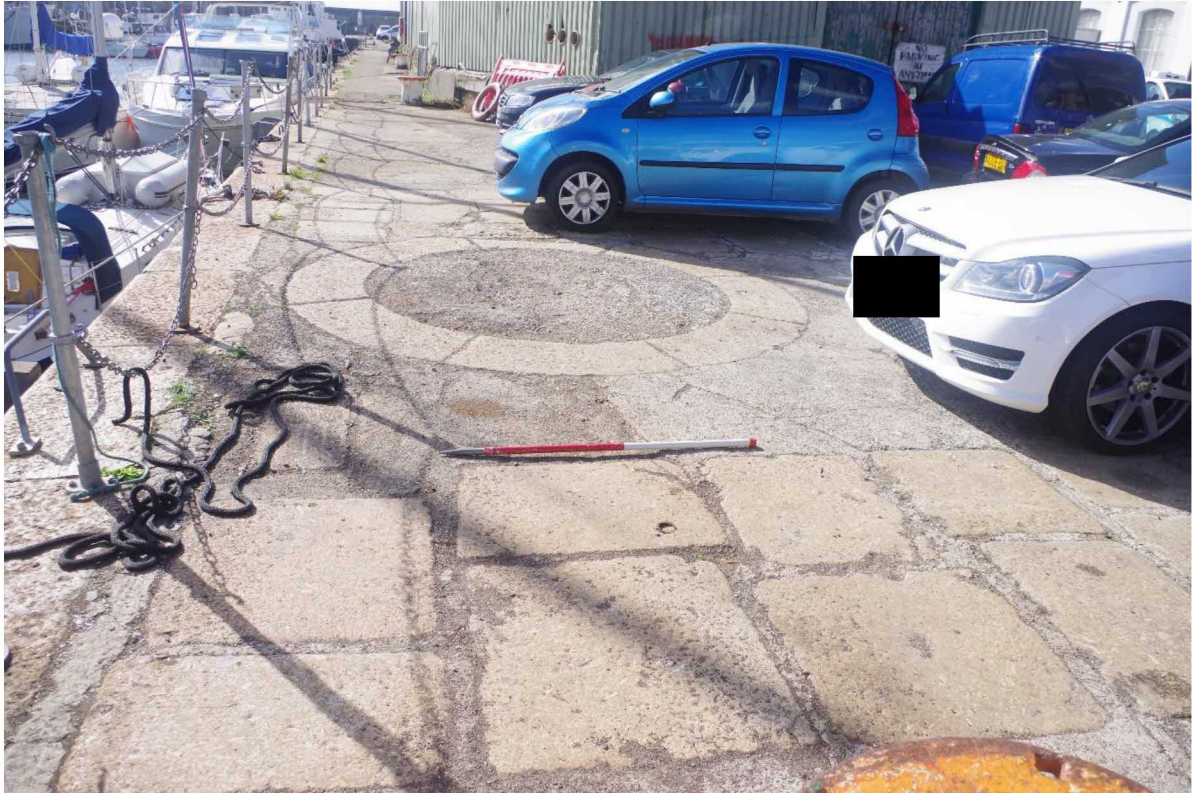
Fig 30 Granite paving and probable tram turntable base adjacent to derrick dating to c1880 (Site 31).
