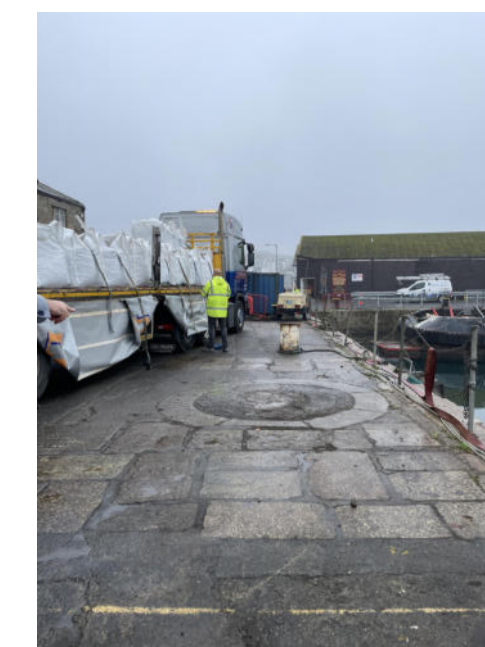
Fig 1. NDHA Granite pavers - tram turntable
