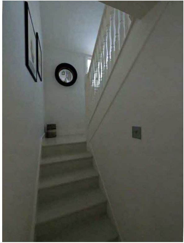
Photo 48 (44) GF to FF stairs from west
