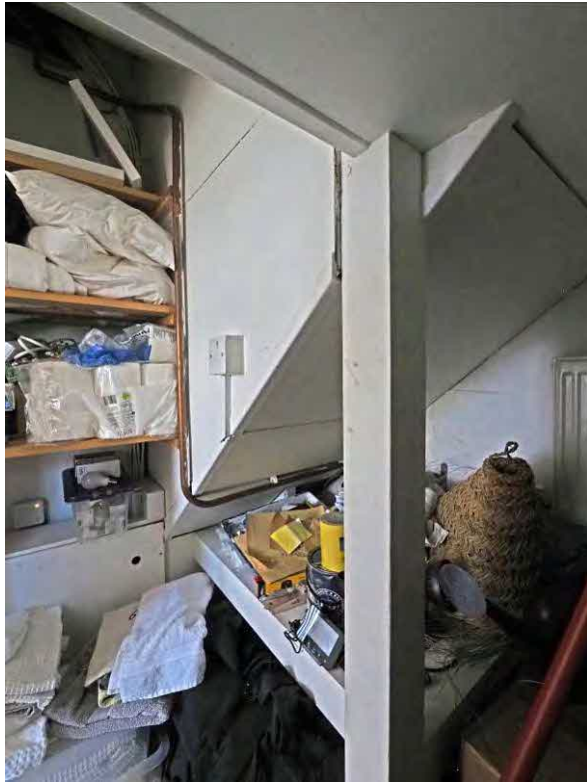
Photo 47 (41) GF under stair from east
