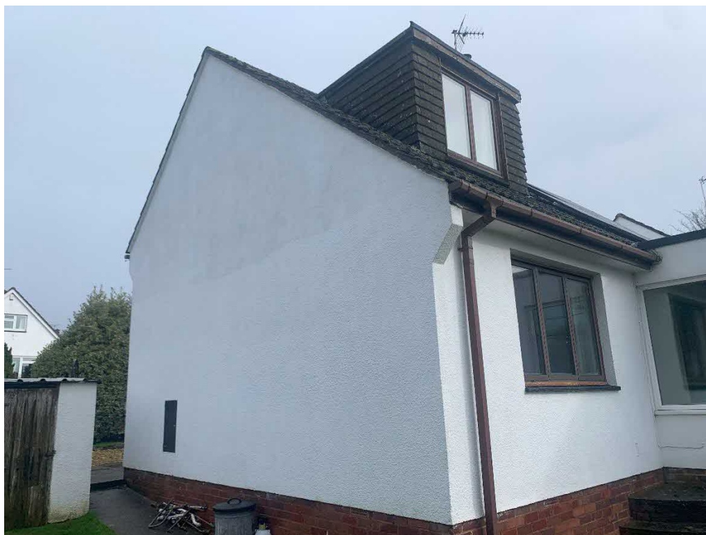
Photograph 1: Existing western gable end of 1 Great Close, Culmstock property.
