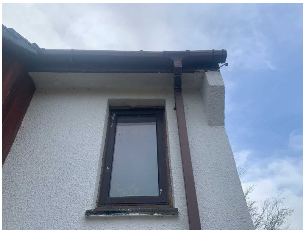
Photograph 2: Typical wall-top detail showing well-maintained nature of the property and lack of potential ingress for wildlife into property.
