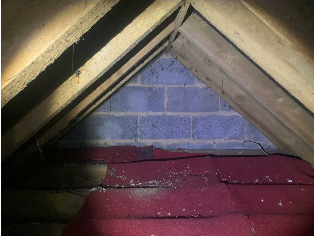
Photograph 3: Internal view of loft space showing low ridge height.
