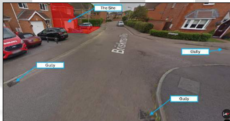
Figure 3-3: Highway drainage gullies
