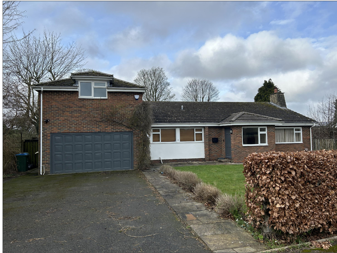
P1 - View from Dove Tree Close
