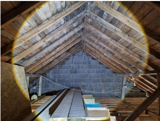
Photo 1: Interior loft of bungalow
