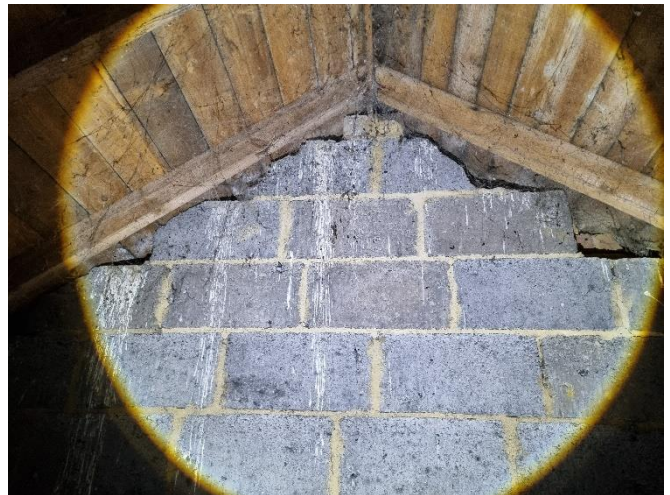
Photo 2: Interior loft of bungalow
