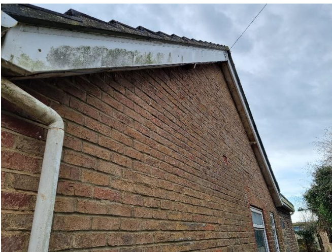
Photo 9: West facing elevation
