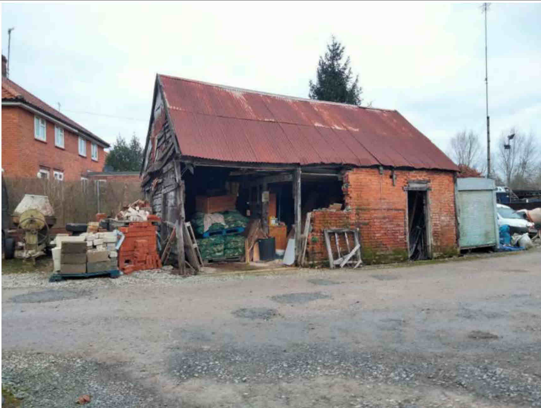
Photo 2 – Southeast elevation of the barn.
