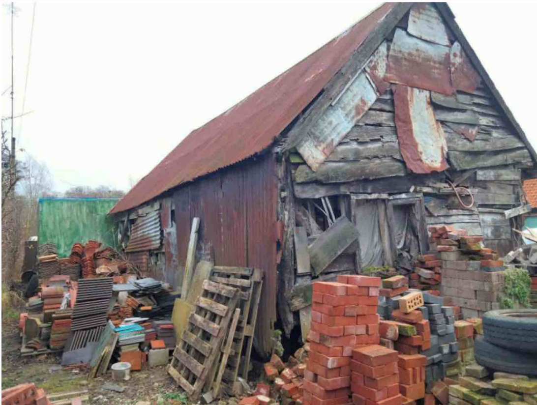
Photo 6 – Reclaimed clay roof tiles stored behind the northwest elevation of the barn.
