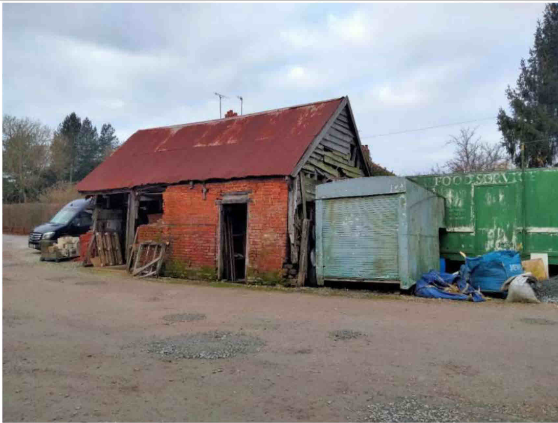
Photo 3 – Southeastern and northeastern elevation of the barn.
