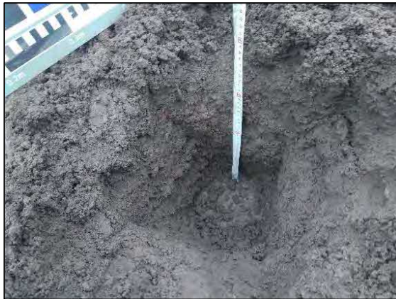
Photograph 5 - VP03, soil depth of 0.42 m. Geotextile visible at the base.
