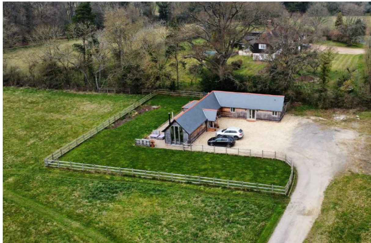
SIDE/FRONT ELEVATION OF EXISTING PROPERTY FROM DRIVEWAY APPROACH
