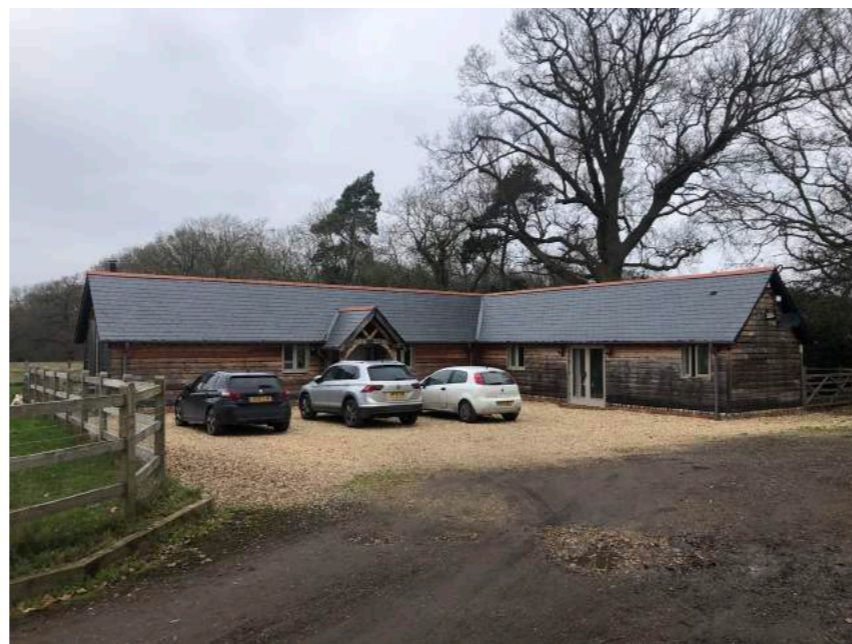
FRONT ELEVATION OF EXISTING PROPERTY
