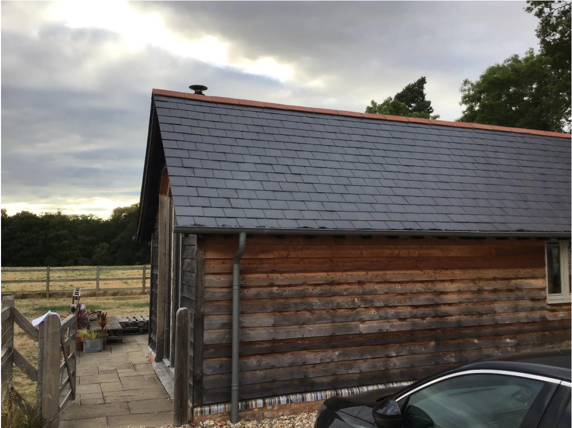
Figure 1. Eastern elevation of South wing of dwelling looking west.
