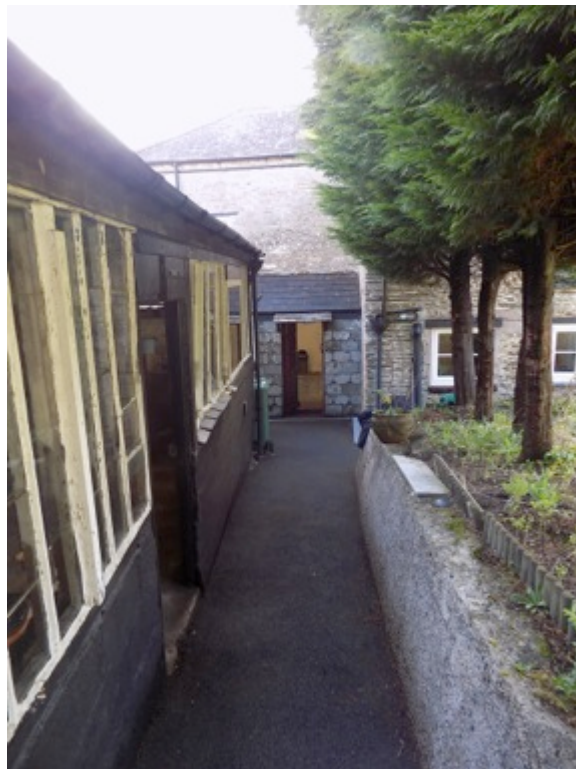
Photo 4. Outbuildings garden(west) elevation, half glazed in timber frame.
