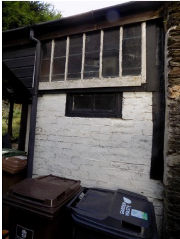
Photo 3. The outbuilding south end a mix of painted brick and timber frame for the W.C enclosure under the hipped slate roof.
