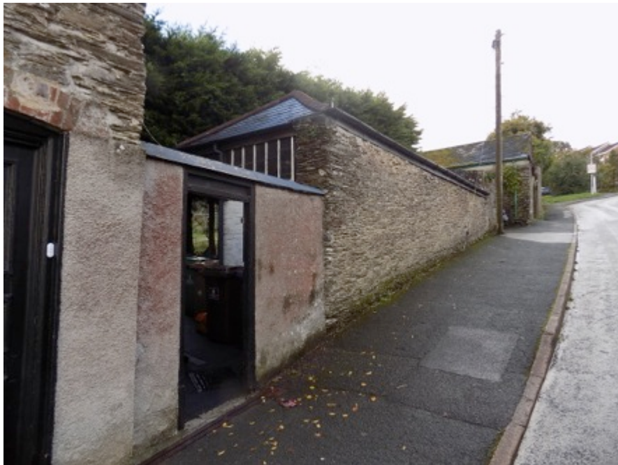
Photo 2. The outbuilding at 'Jessops' onto Horsham Lane. Linked by a section of garden wall with timber board gate that provides rear access of the property.
