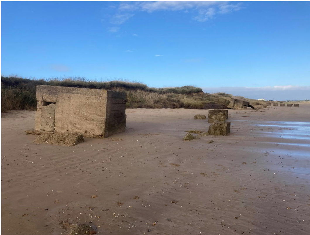
Photograph 1: View of landfall from the south. The planning application boundary passes between the anti-tank blocks (MHU21031) and the pillbox (MHU21027) in the distance.
