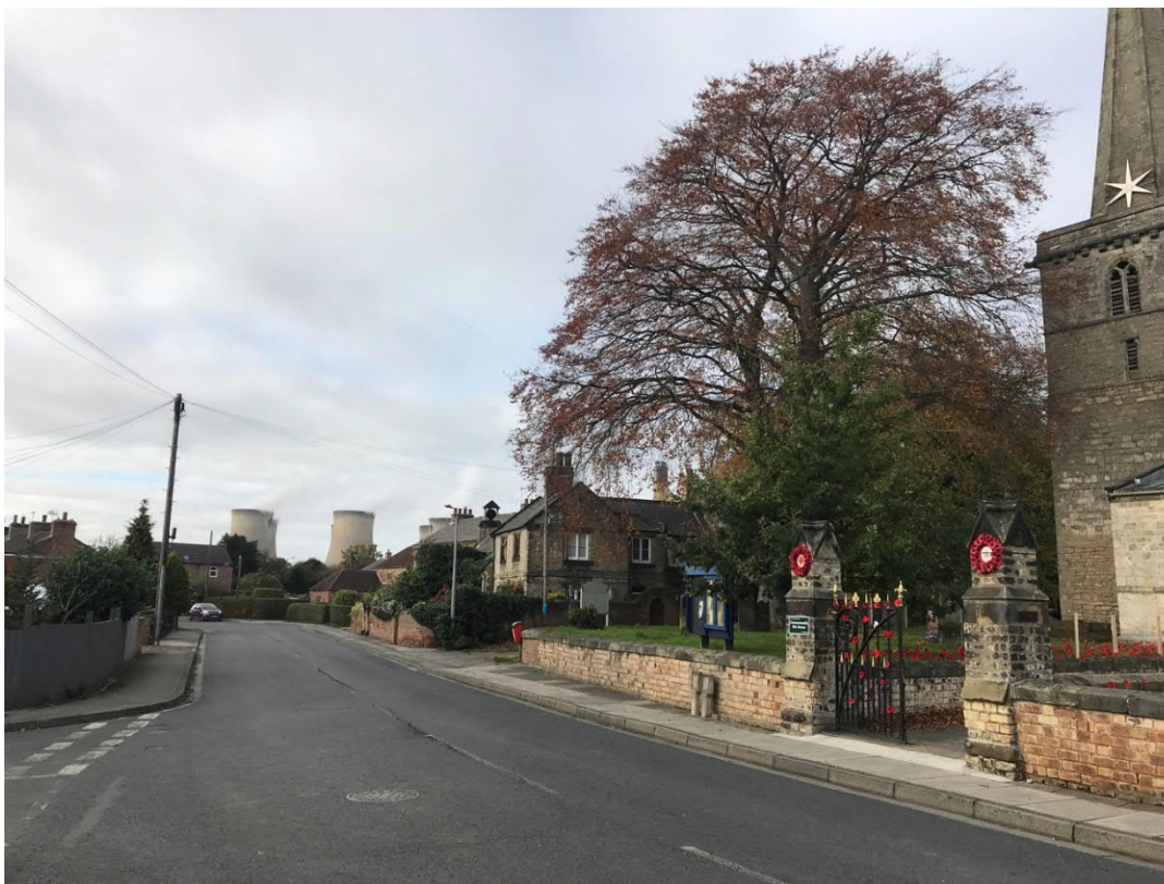
Photograph 24: View towards Drax Power Station from Drax Village outside of the Grade I listed Church of St Peter and St Paul (LB1148397).
