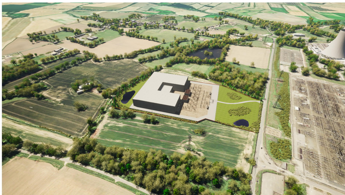
Figure NTS-5: Indicative image (looking from the north) of the proposed converter station
