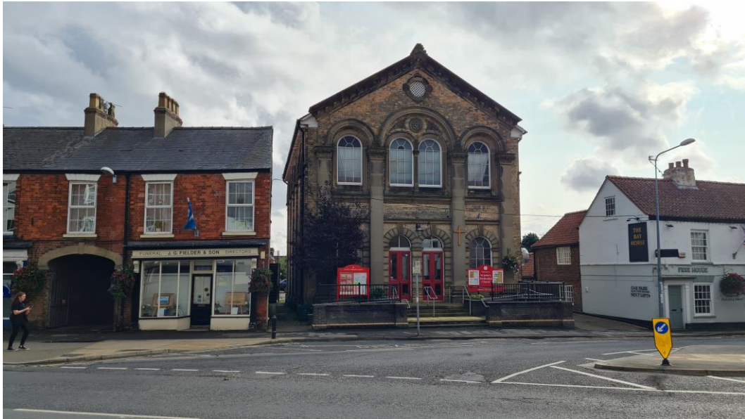
Figure 4 St John Methodist Church, Front Elevation and entrance on Market Place, Market Weighton
