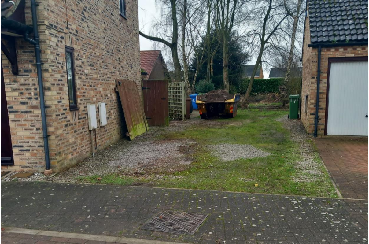
A – showing entrance/access to the site (land to the rear of 45 West End, South Cave) looking south west (from West End Farm Close)
