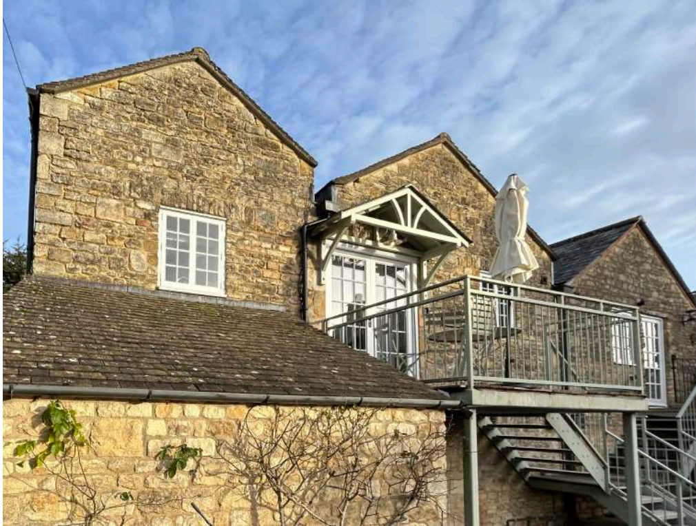
Photo 3 – showing canopy roof as installed – note external light over doors
