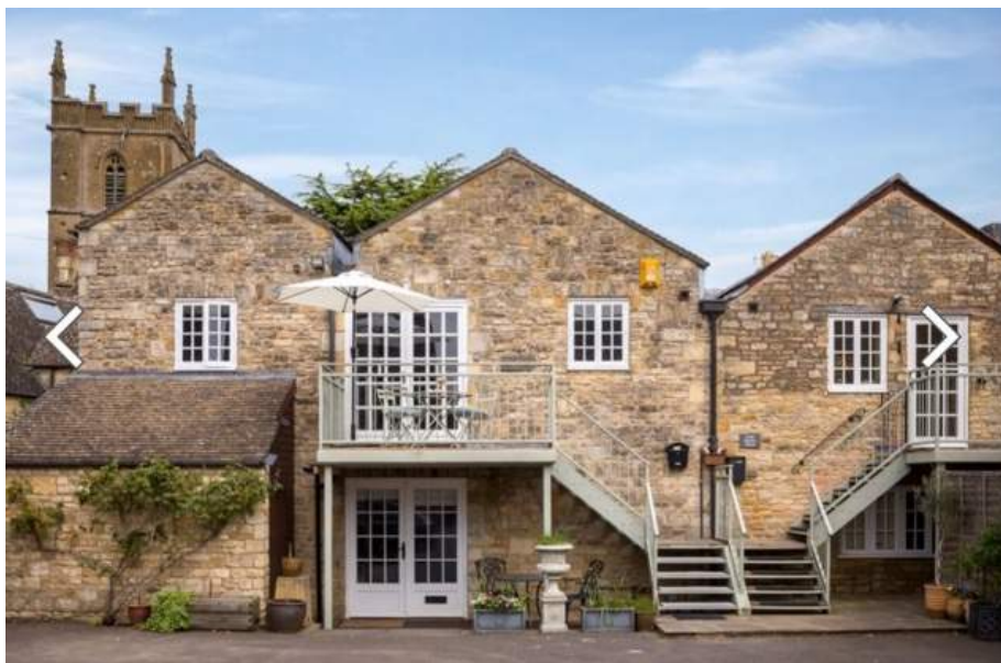
Photo 1 – taken prior to installation of canopy roof
