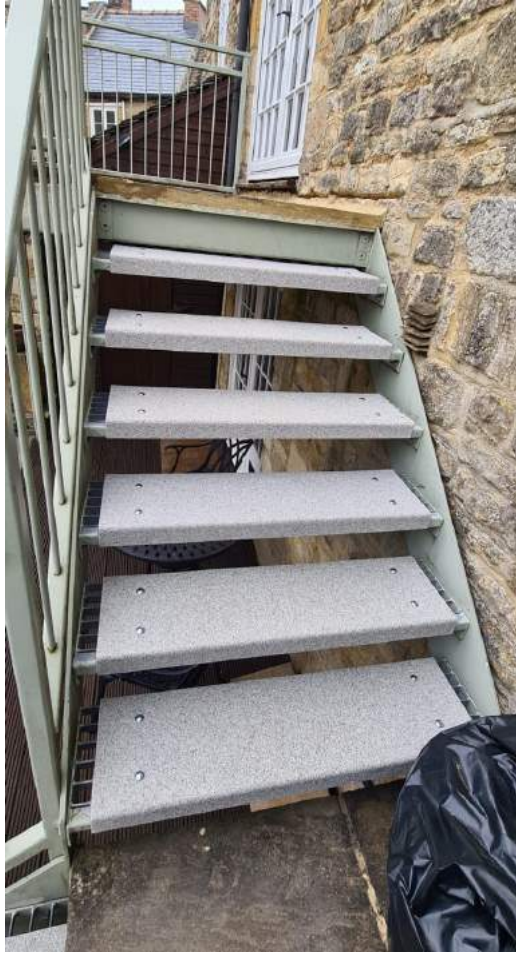
Photo 4 – showing non-slip treads and edge of slate to stair landing
