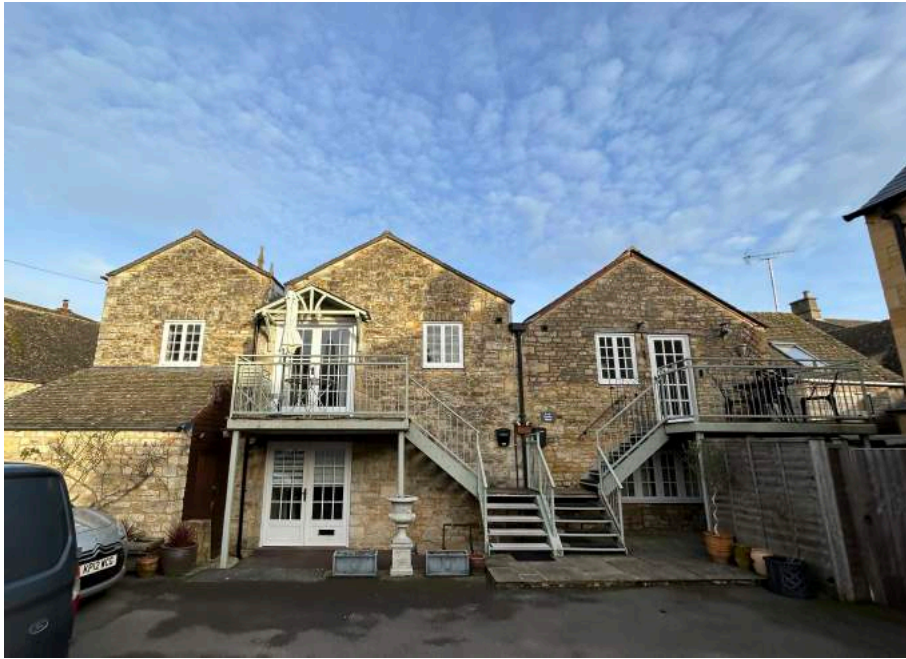
Photo 2 – taken after installation of canopy roof
