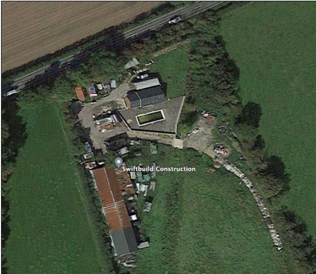
Figure 10- Aerial image of the site from 2020 (Source- Google Earth Pro).
