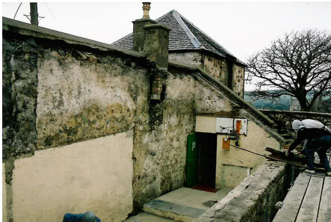
Rifle range interior looking south following roof strip, 2003
