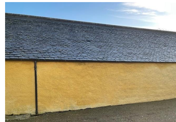
Cast iron rainwater goods
