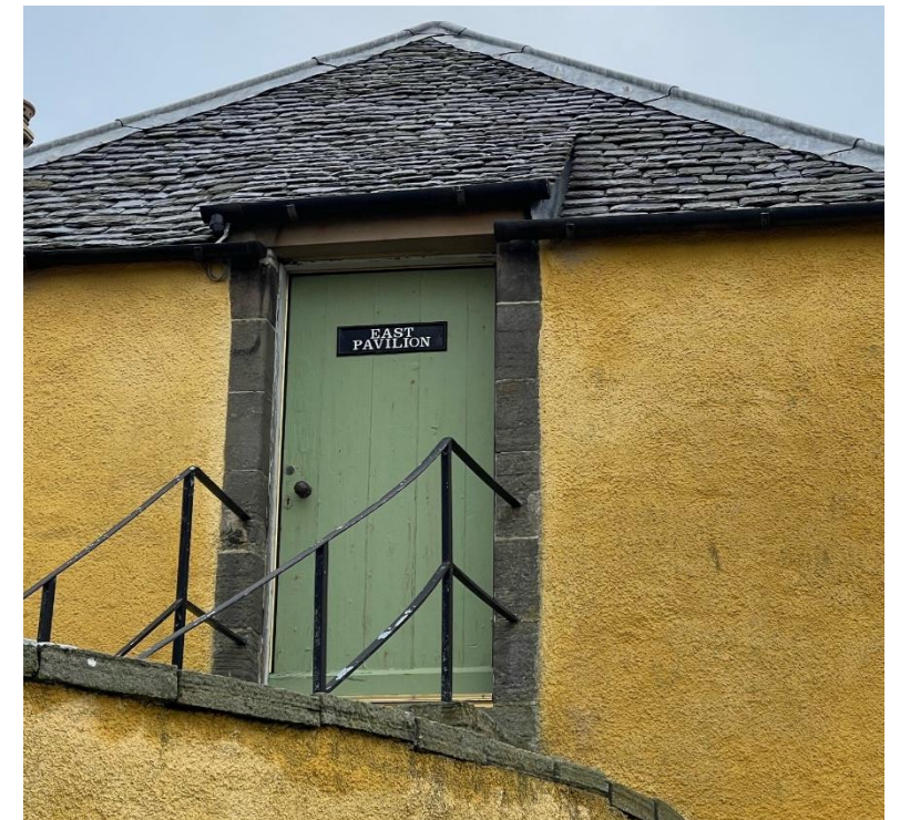
Existing Raised Lintel Detail
