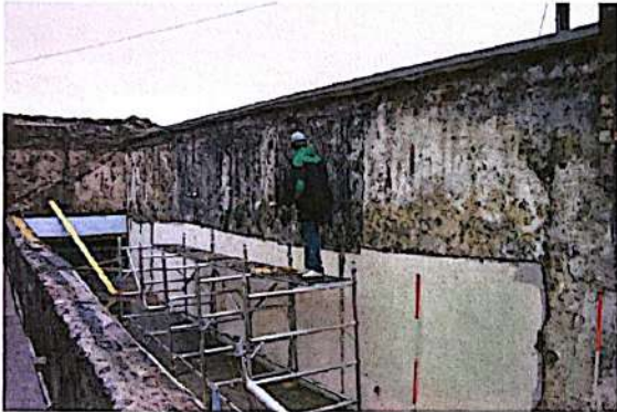
Photograph 1 – E wall, looking N.
