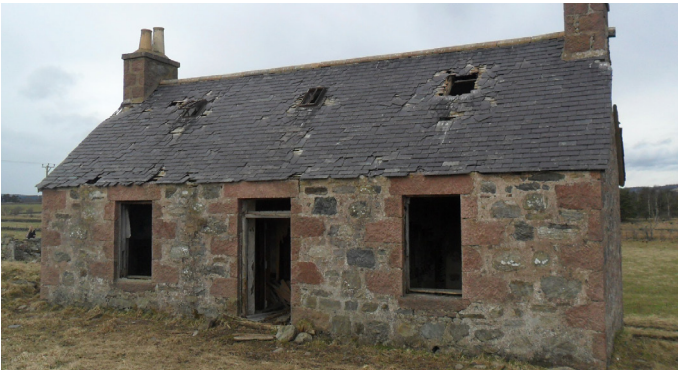
Existing Building- The Bothy - South Elevation
