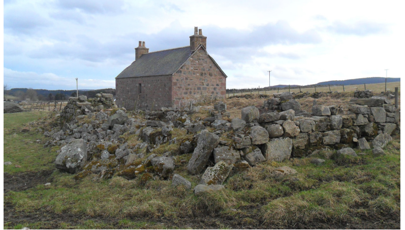
Viewing North West towards The Bothy
