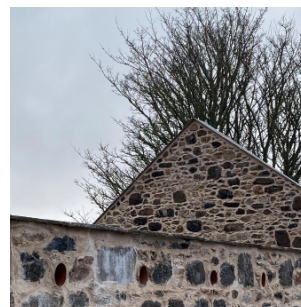
Existing stone walls (re-pointed)
