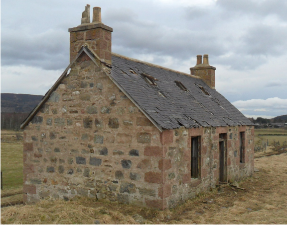
Existing Building - The Bothy - South and West Elevation
