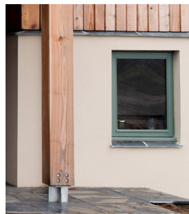
Timber and steel post
