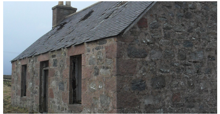
Existing Building - The Bothy - North and East Elevation
