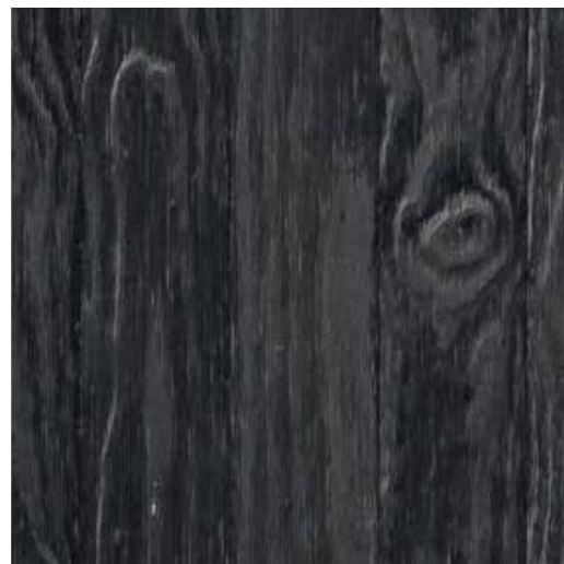
Timber - Walls lower level
