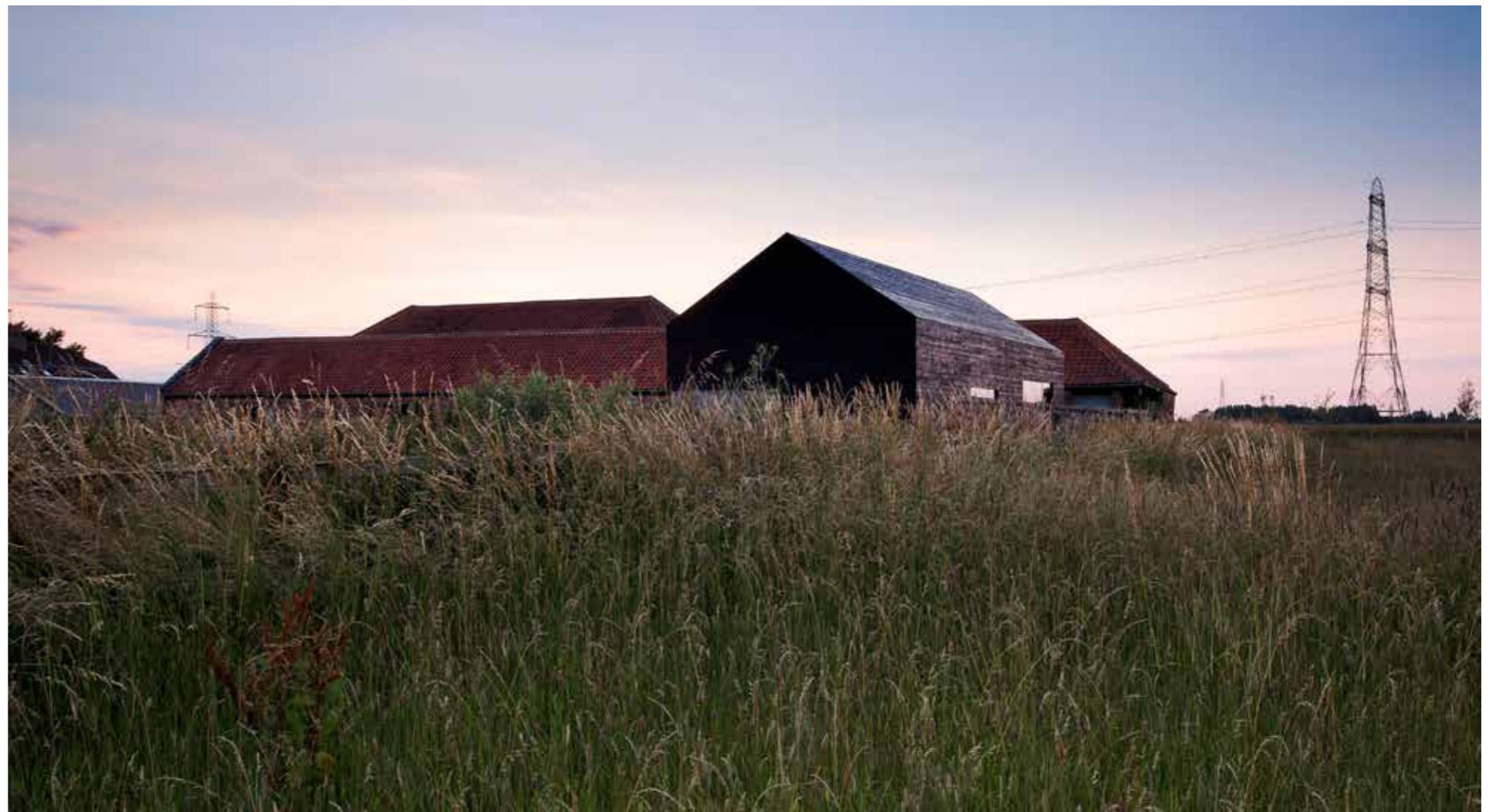
Precedent of new dwelling house at a Cambridgeshire farm: an un-ornamented black-clad volume.
