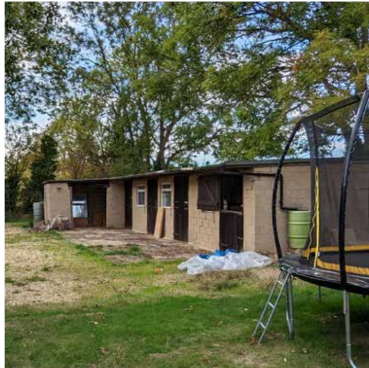
Existing Stable Block
