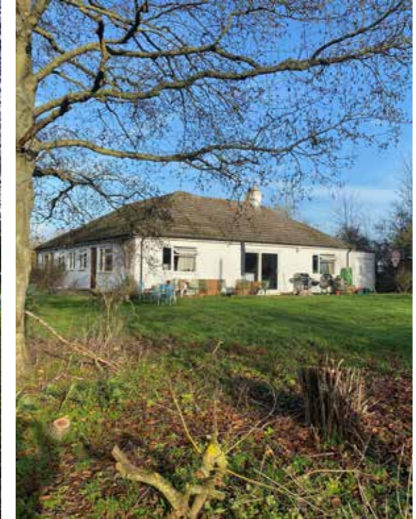
View of Southern Elevation of House
