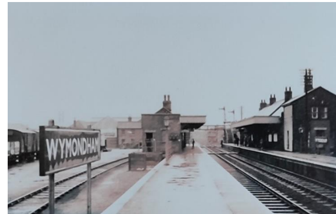
Above Towards Wymondham Station from Norwich : After canopy reduction (Note rendered station building wall)
