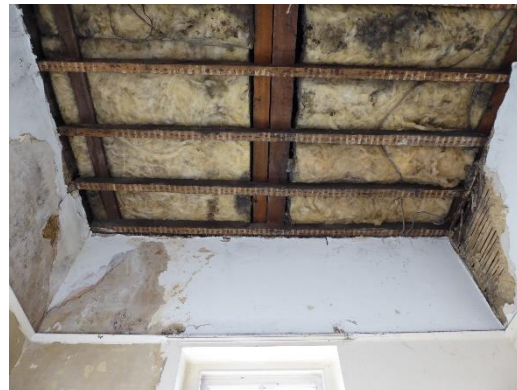
Above Ceiling Post strip-out. Photo 5.
