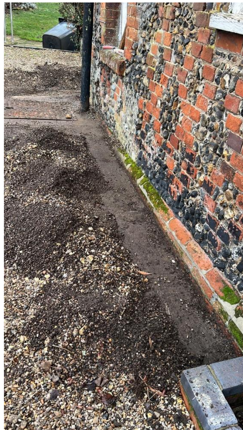
Above Reduced ground level : Front Elevation
