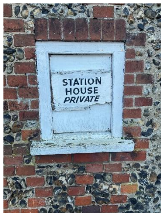
Above Front Elevation Window and brickwork 'diapering' within 'knapped flint'
