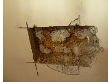
Above External wall trial hole. Photo 3.
