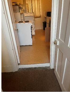
Above Kitchen Pre strip-out. Raised floor. Photo 1.
