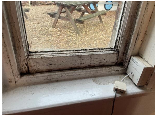
Above Photo 5 (Window WG-2 Pre Strip-Out)
