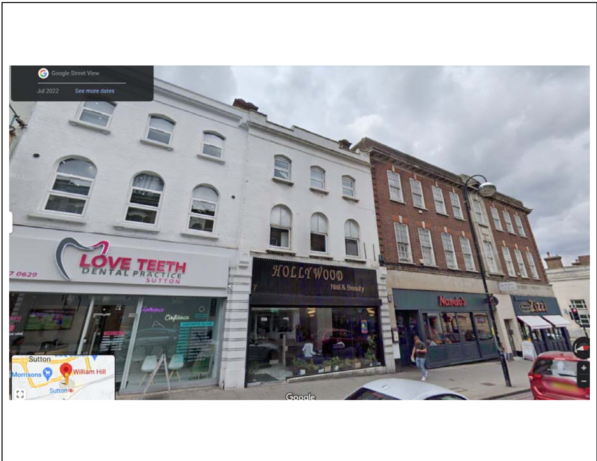
8. High Street Streetscene – showing adjacent PVC windows
