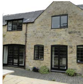
1990's timber framed double glazing replaced with PVC-U in a more appropriate design and traditional colour to enhance the property.
