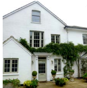
Not all sash windows are white! Before the late Victorian period a much wider range of colours were originally used.
