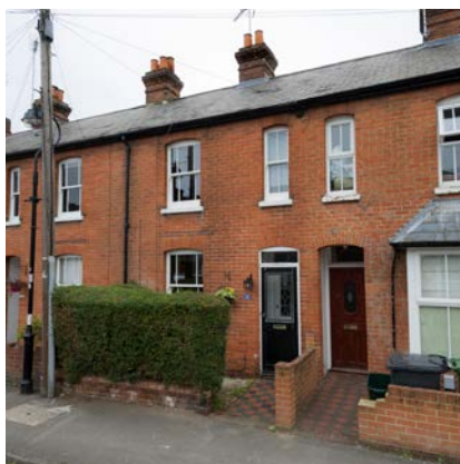
Brook Street Conservation Area — after installation to the middle property
