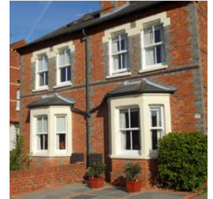
Wood stained timber framed top-hung casements (installed some 30years ago) were replaced with sliding box sash. (Mansfield)
