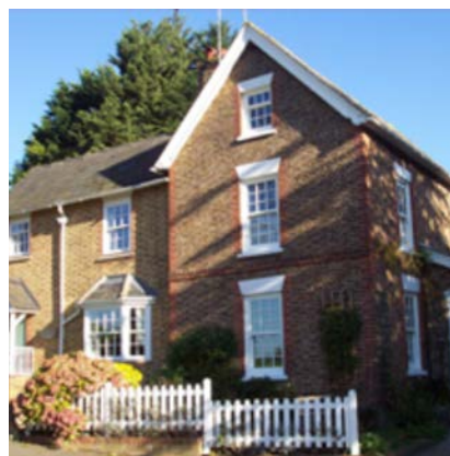
New PVC-U windows alongside some original timber windows in the front of this property (near Maidstone, Kent)
