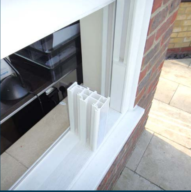
Attention to detail and innovation to meet challenges – To overcome a Conservation Officer's objection to the exposed stop end detail, the Masterframe technical team developed an internal item that would not be visible.
