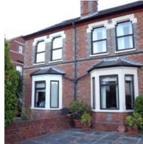
Wood stained timber framed top-hung casements (installed some 30years ago) were replaced with sliding box sash. (Mansfield)
