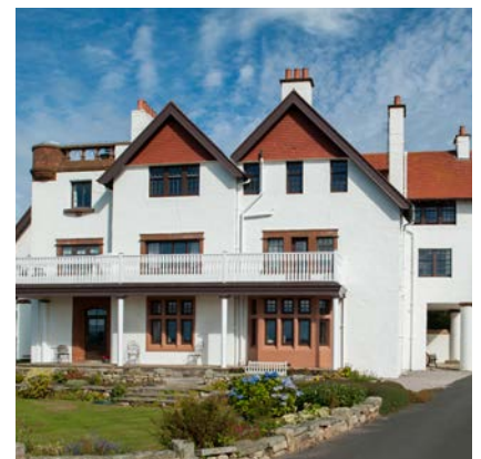
Replacement using Vintage Traditional windows in the flats at Mokoia House, Troon. Locally approved – “rigorous levels of quality and detailing”.
