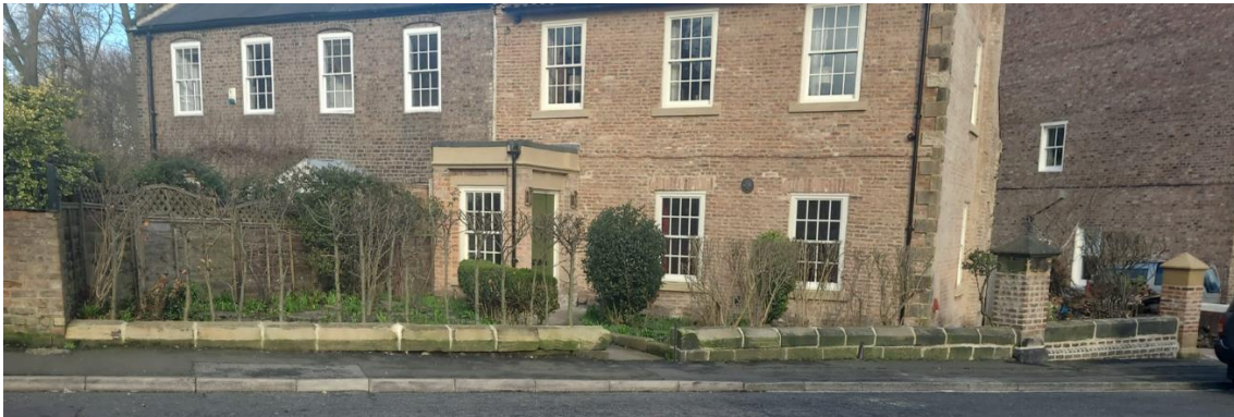
Figure 1 – Cross House Without Railings
