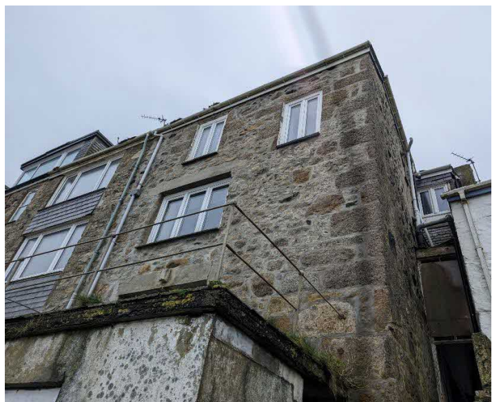
Photo 2. Showing the house from the rear (north)
