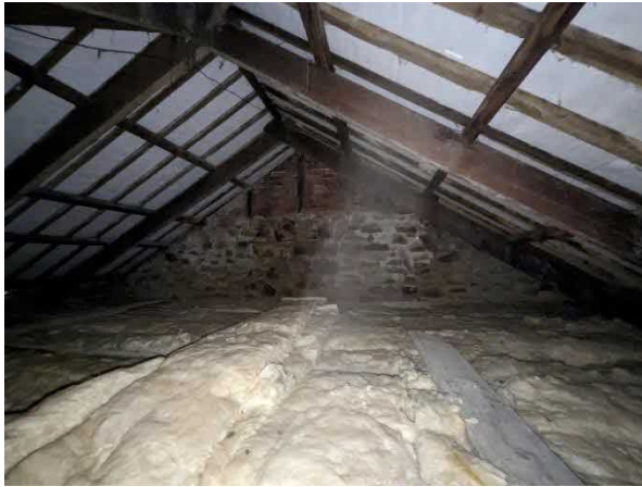
Photo 3. Showing the roof void looking east
