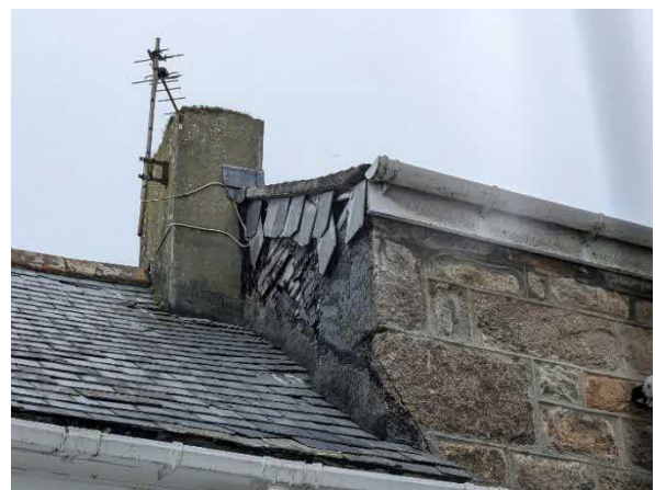
Photo 6. Showing the western gable end
