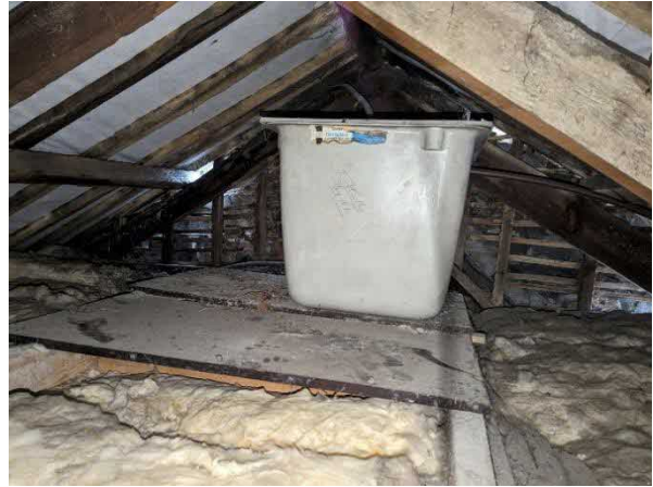
Photo 4. Showing the roof void looking west
