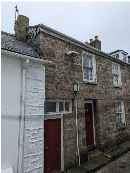
Photo 1. Showing the house from the front (south)
