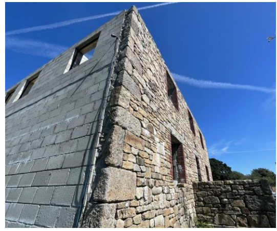
Figure 4. West and south elevation
