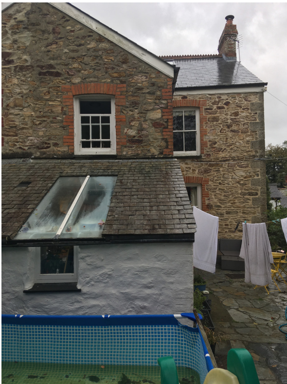
Fig.1 photograph of the rear elevation with small lean-to in the foreground
