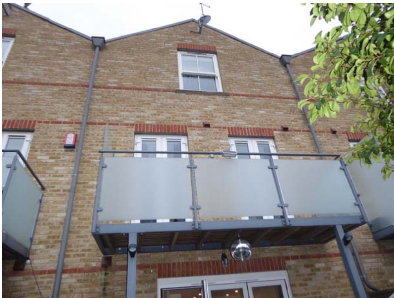
Fig 1: Existing rear elevation
