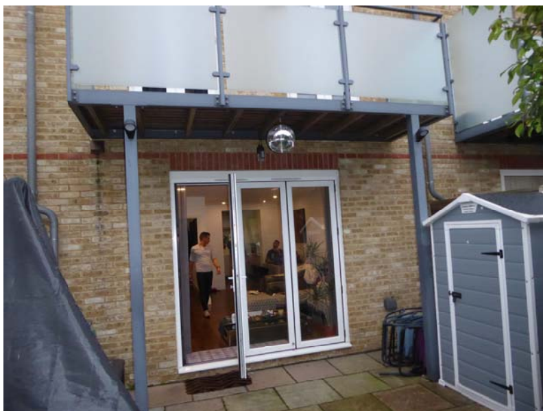
Fig 2: Existing ground floor aluminium-framed bi-folds door to be repurposed and installed at first floor level
