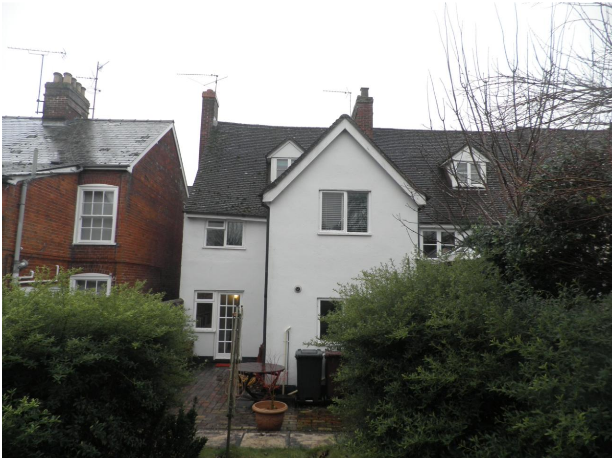
Photograph of Existing Rear Elevation
