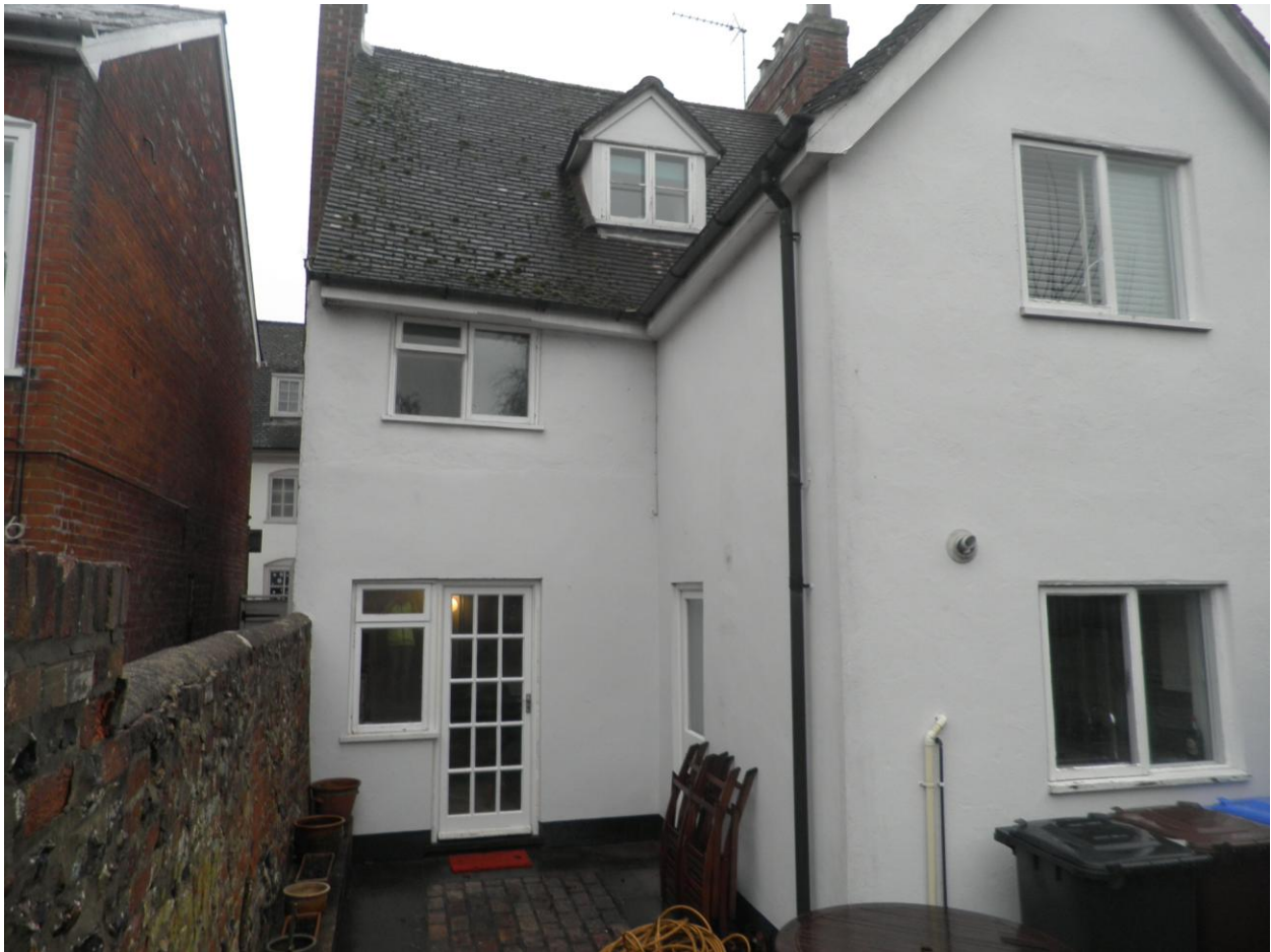
Photograph of Existing Rear Elevation
