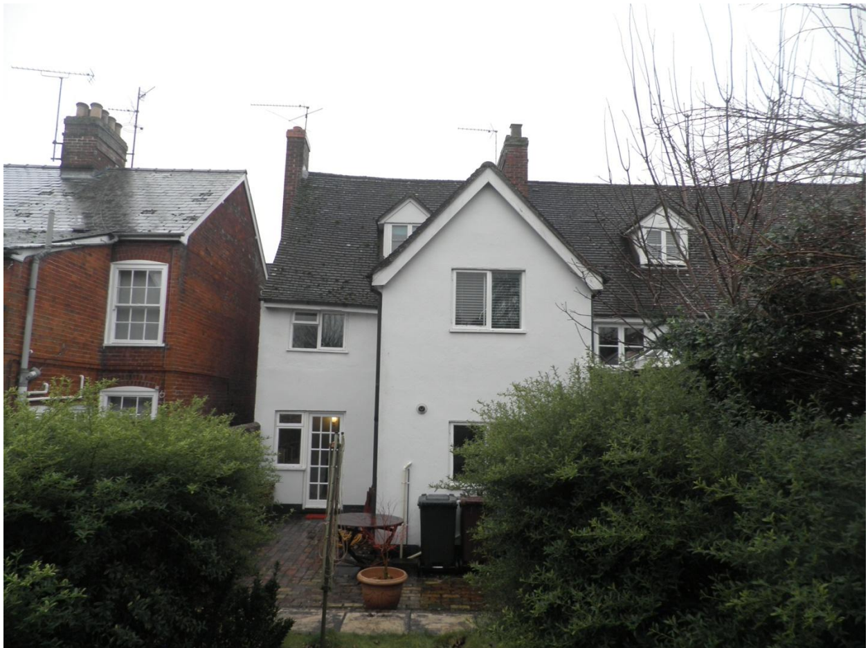
Photograph of Existing Rear Elevation
