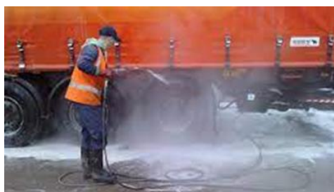
Wheel Cleaning Prior To Leaving Site
