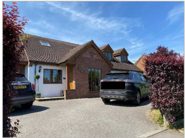
Conservation Area: Modern bungalow mixed render and brick finishes
