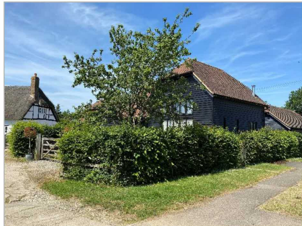
Conservation Area: modern barn-style single dwelling
