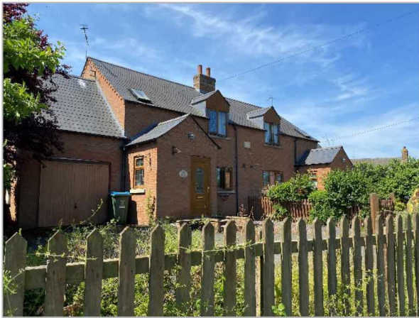
Conservation Area: Modern two storey road-facing, monolithic brick finish
